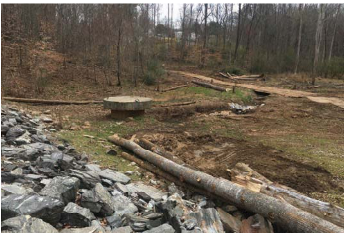
Greenwood Pond Constructed Wetlands
