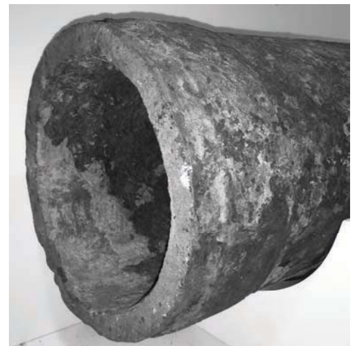
1829 7" Cast Iron Water Line (Sections are still in service)
