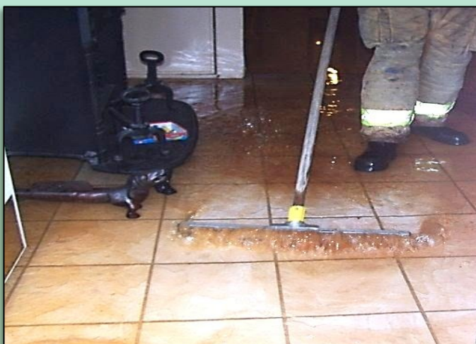
Water main break – flooding of private property.
