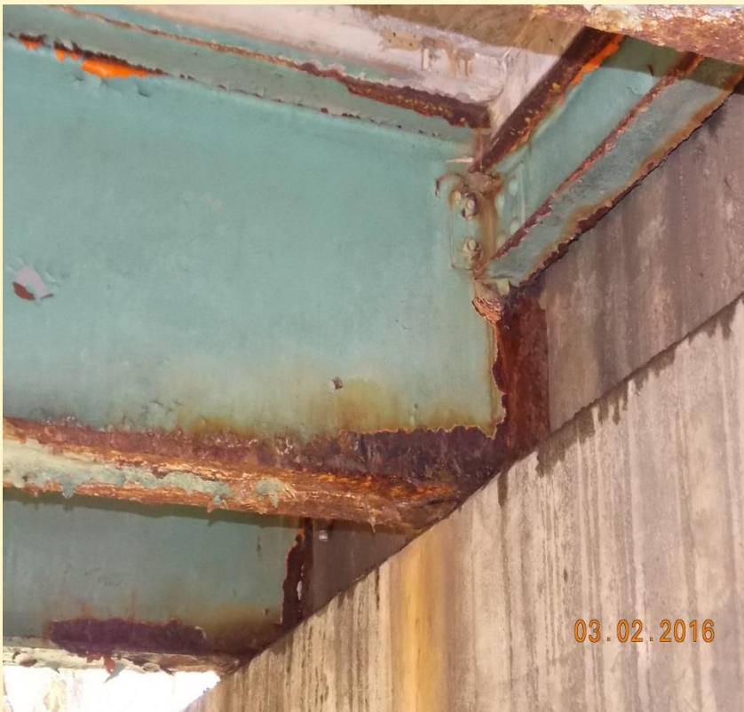
Link Road Bridge Beam
