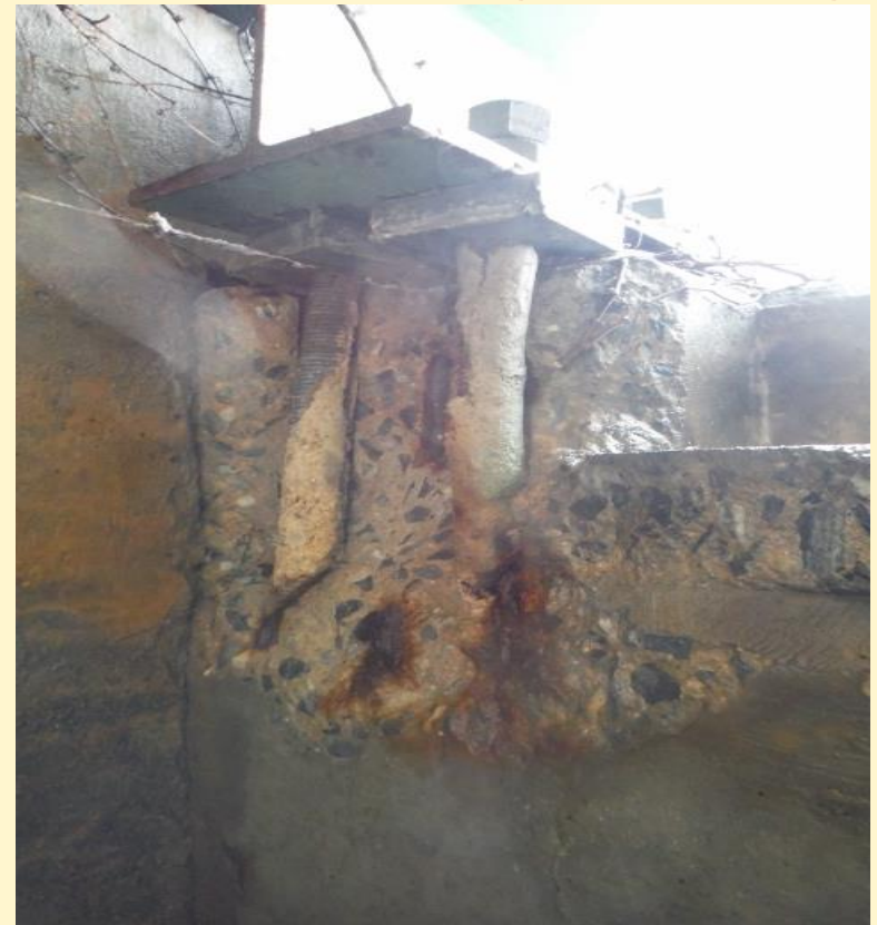
Link Road Bridge Railing
