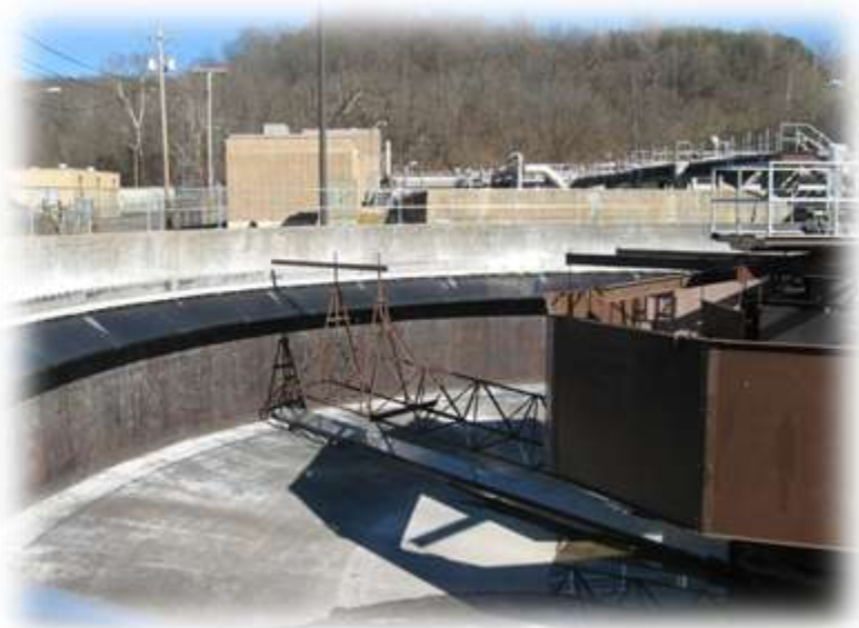
RWWTP Secondary Clarifier
