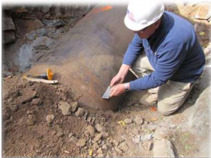
Corrosion engineer making pitting measurements.
