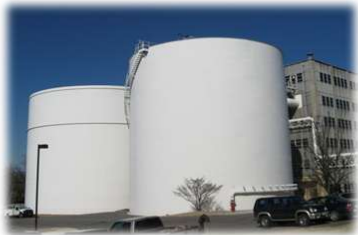
College Hill Coagulation Tanks
