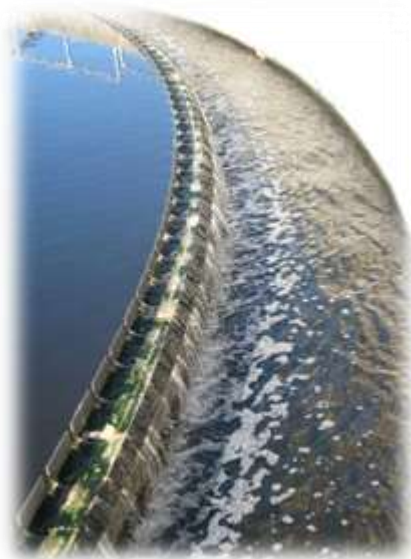
RWWTP Secondary Clarifier
