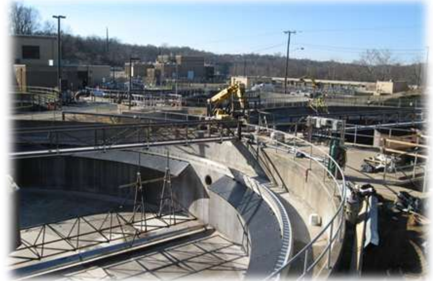
RWWTP Secondary Clarifier
