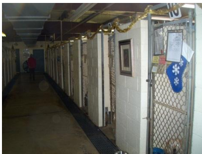
Graphic #24 – Trench Drain Location
