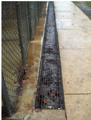
Graphic #2 – Exterior Trench Drain
