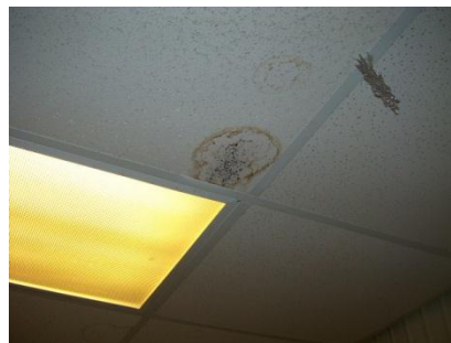
Graphic #9 – Roof Leak
