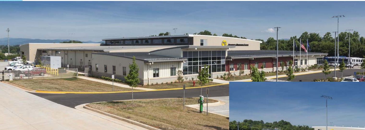
Operations & Maintenance Facility
