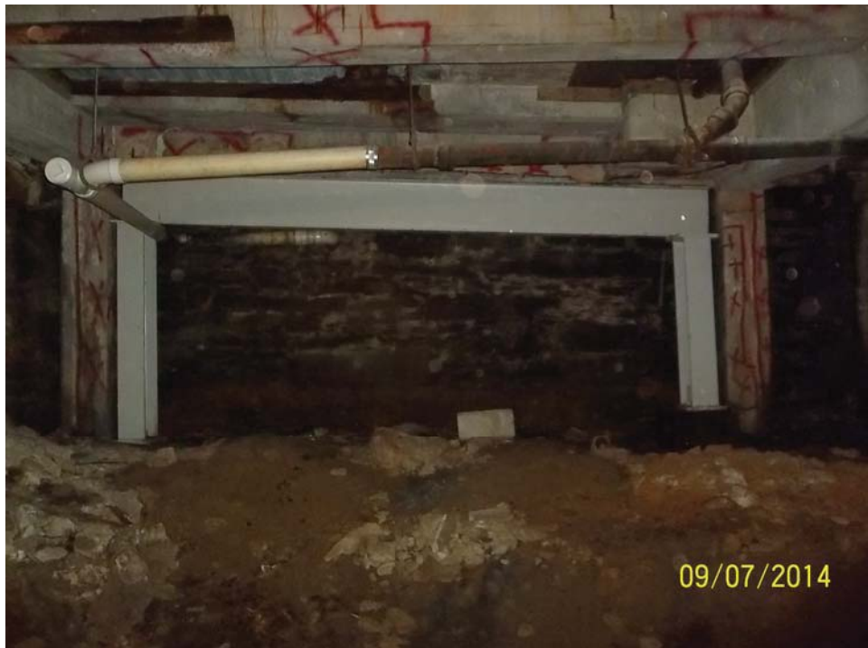
(22) Bay B panel 1 – Temporary bent at entrance
