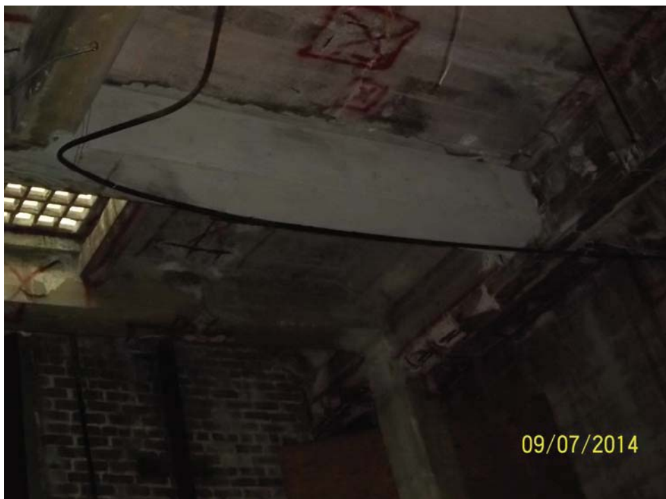
(27) Bay D panel 9 – Concrete beam repair
