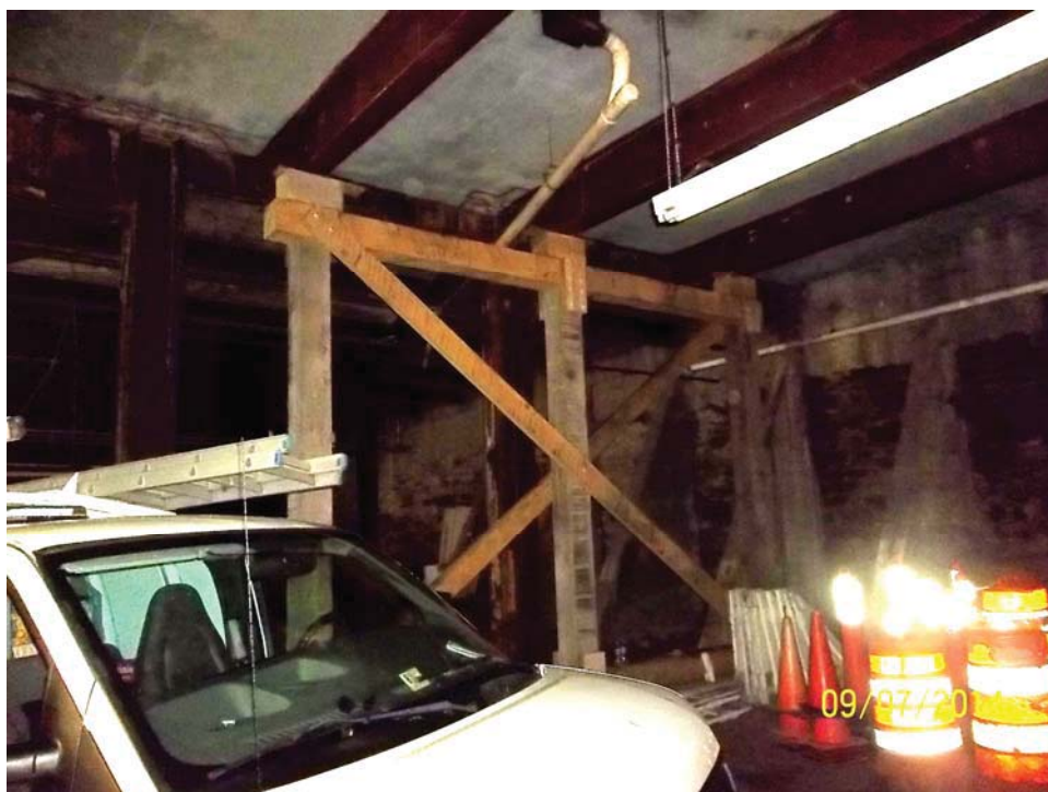
(16) Bay A1 & Bay B panel 10 – Timber bent
