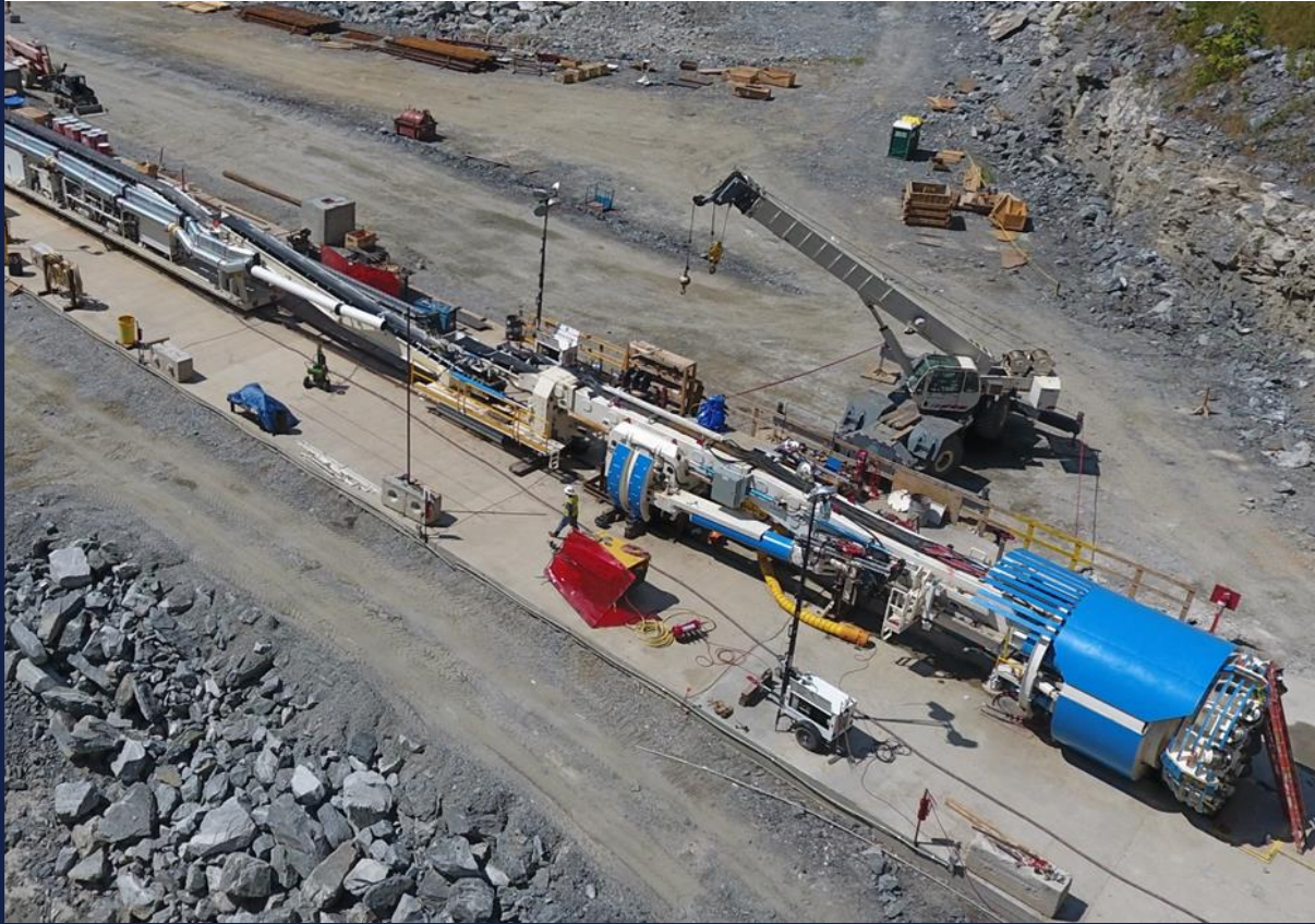
Tunnel Boring Machine (TBM)
