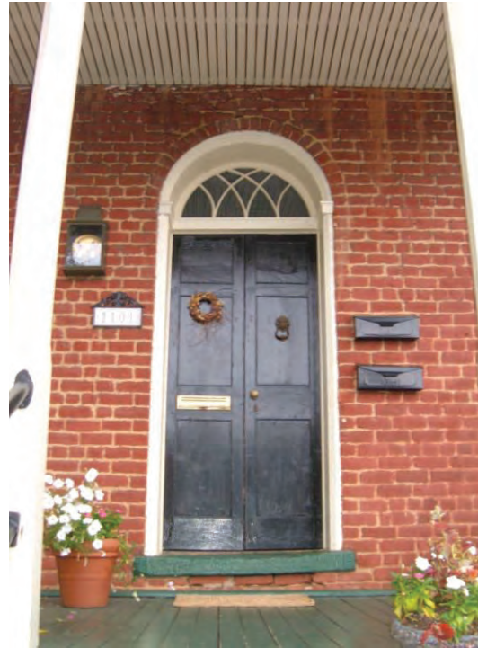
Federal style door at 1101 Jackson Street.
