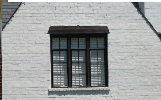
Original steel casement windows of the 20 th century should also be repaired as needed and retained.
