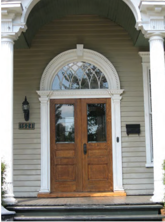
Doors are often character defining features such as this Colonial Revival door at 1524 Rivermont Avenue.
