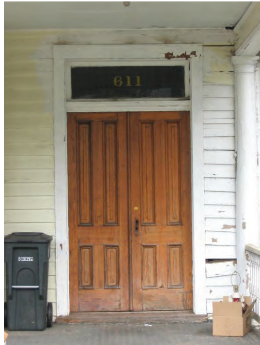
Original paneled wood doors at 611 Washington Street.
