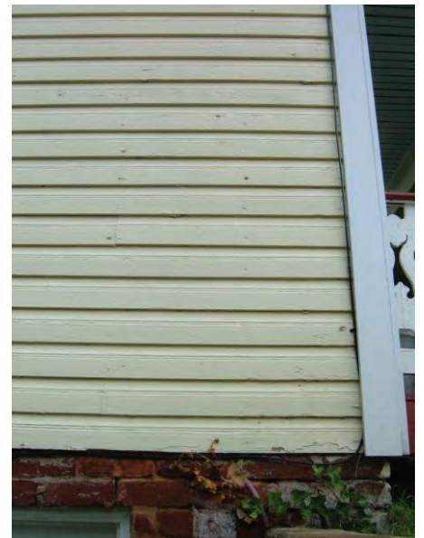
Original wood siding at 1000 Harrison Street.
