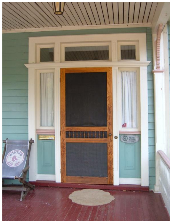
Replacement screen doors should be of the appropriate period of the building (118 Madison Street).
