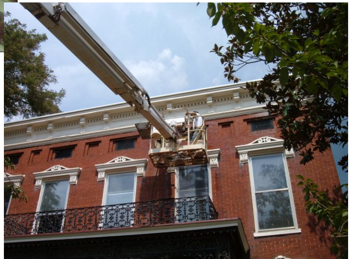
Masonry should be cleaned with water and detergents or chemicals (818 Court Street).
