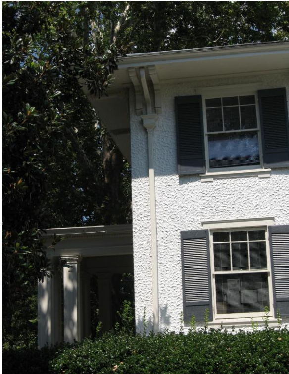
Box gutter and downspout at 2208 Rivermont Avenue.
