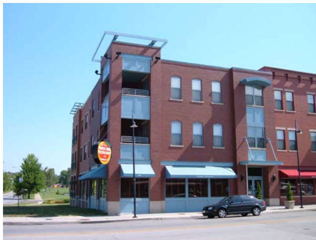
This new building effectively uses both historic elements like arched windows as well as contemporary touches in the recessed corner bay.
