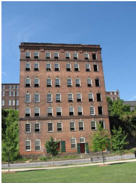
Building in the 1300 block of Jefferson Street in Lower Basin undergoing rehabilitation as part of the “Lower Bluff Walk” (from the Downtown & Riverfront Master Plan 2000).
