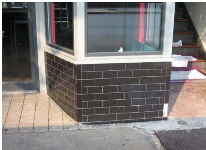
Original tile bulkhead at 1120 Main Street.
