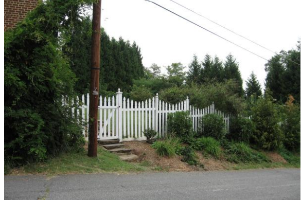
Appropriate privacy fence at 416-418 Washington Street.
