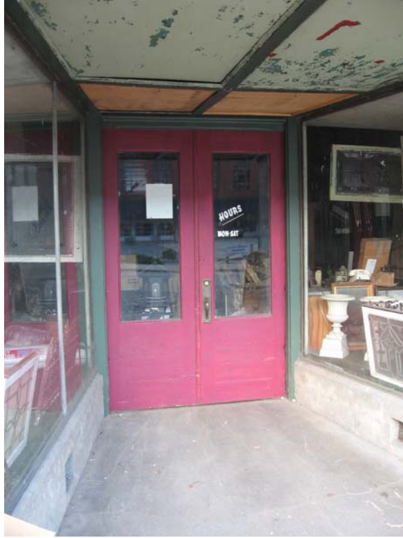
Recessed entrance and original double doors at 1216 Main Street.
