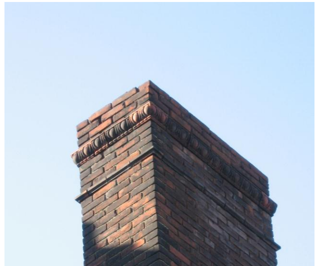
Chimneys were often designed with decorative brickwork such as this egg and dart molding (1022 Court Street).
