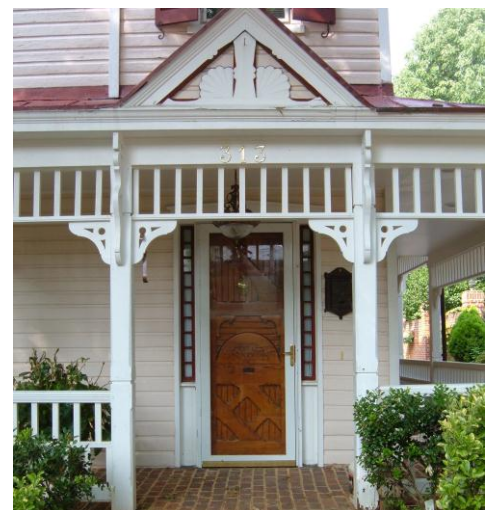
Storm doors should be full view design in order to expose the historic door behind it (313 Madison Street).
