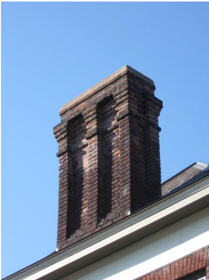
Chimneys should be preserved, maintained, and repointed in accordance with masonry guidelines (1022 Court Street).
