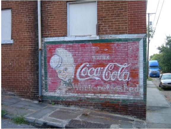
Preserve and maintain original wall signs (508 Cabell Street).
