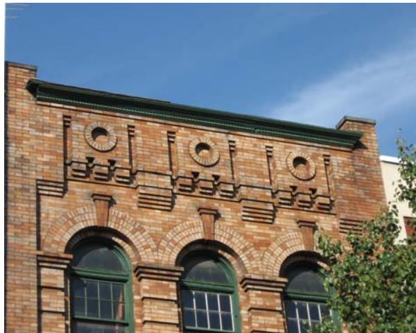
Corbelled brickwork at 909 Main Street.
