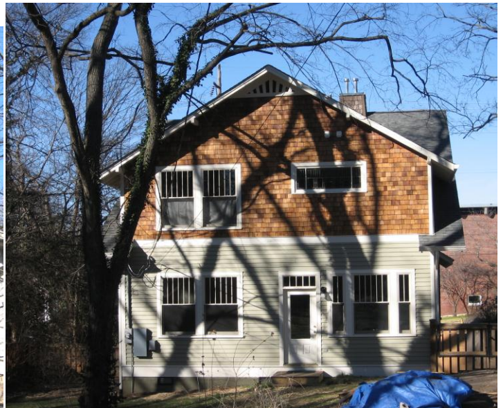
Appropriately scaled rear dormer addition which is recessed from the side gable roofline.
