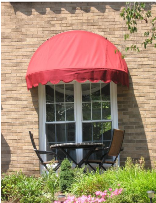
Appropriate use of an arched canvas awning at 2306 Rivermont Avenue.
