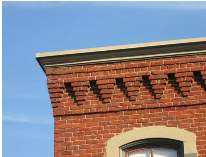
Corbelled brick cornice at 325 12 th Street.
