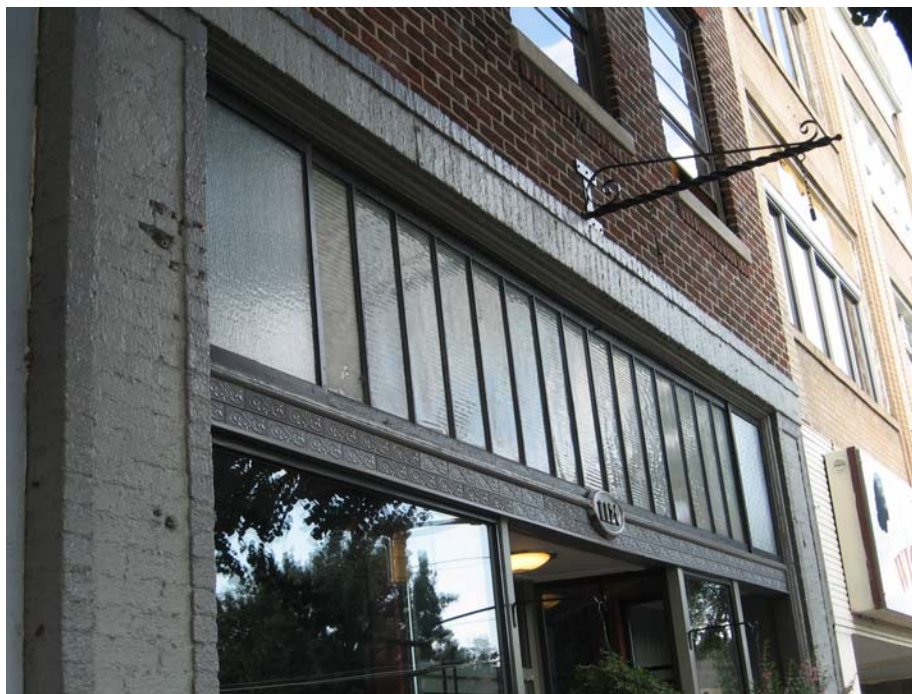
Original divided light transom at 1120 Main Street.
