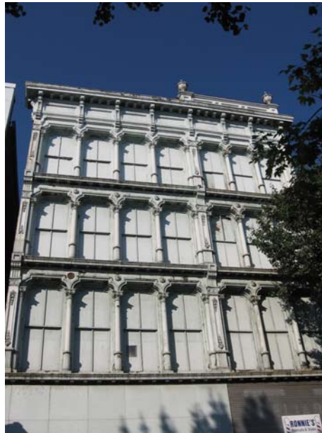
The building at 1021-1023 Main Street has an exterior of cast iron and sheet metal.
