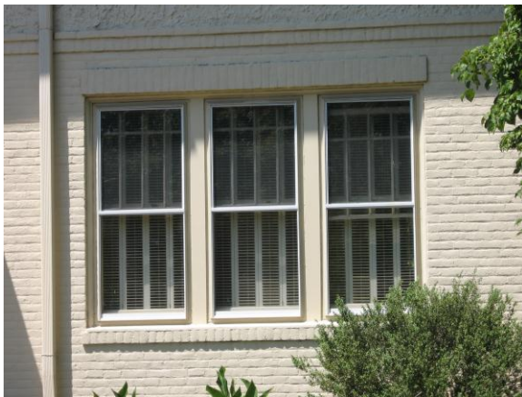
Storm windows should be of full view design or with meeting rails to match the historic window such as at 2460 Rivermont Avenue.
