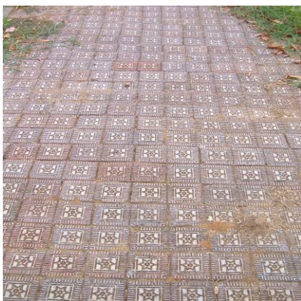
Brick sidewalk pattern in the 900 block of Federal Street.
