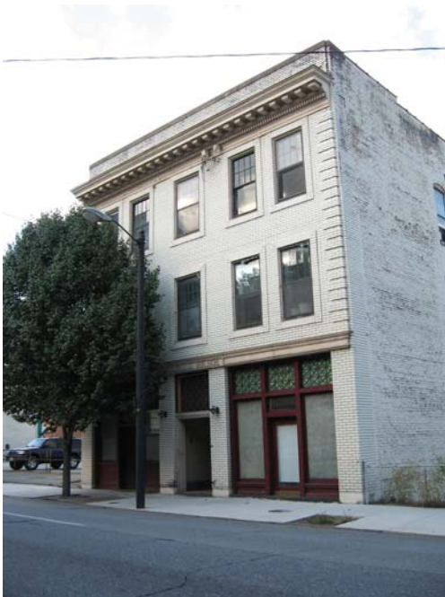
The Professional Building in the 1000 block of Church Street is a restrained example of the Colonial Revival style.
