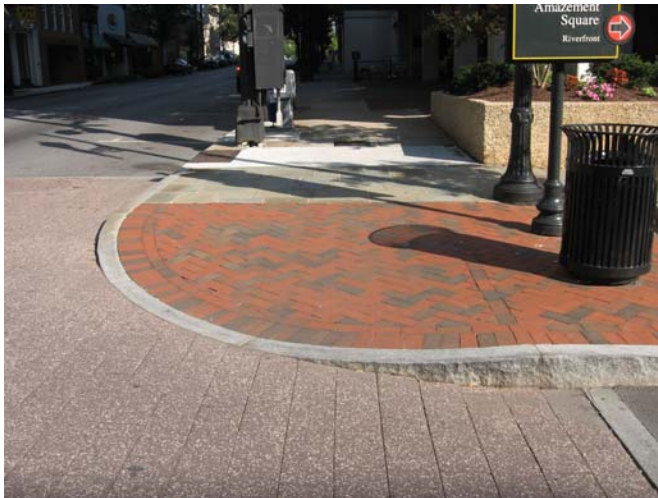
Added streetscape elements including ADA curb cuts, brick sidewalks and street furniture (9 th and Main Streets).
