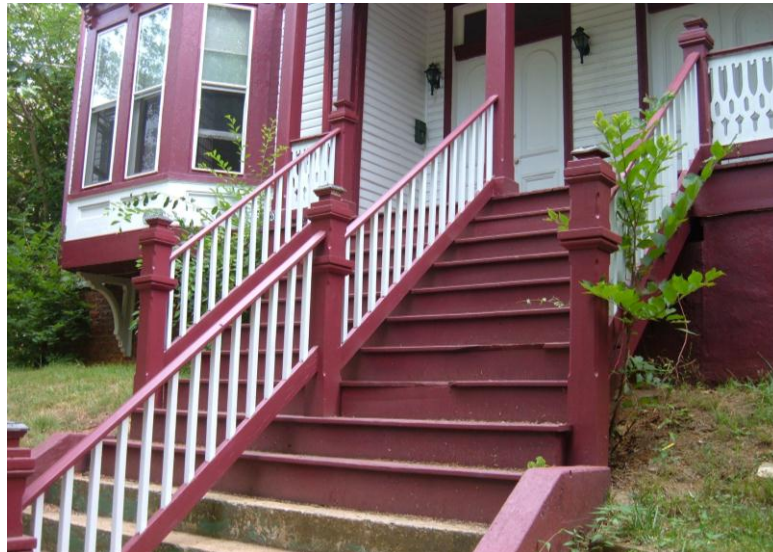
Appropriate rebuilt staircase at 202-204 Harrison Street.
