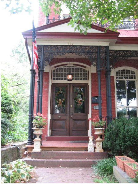
Cast iron porch at 307 Washington Street.
