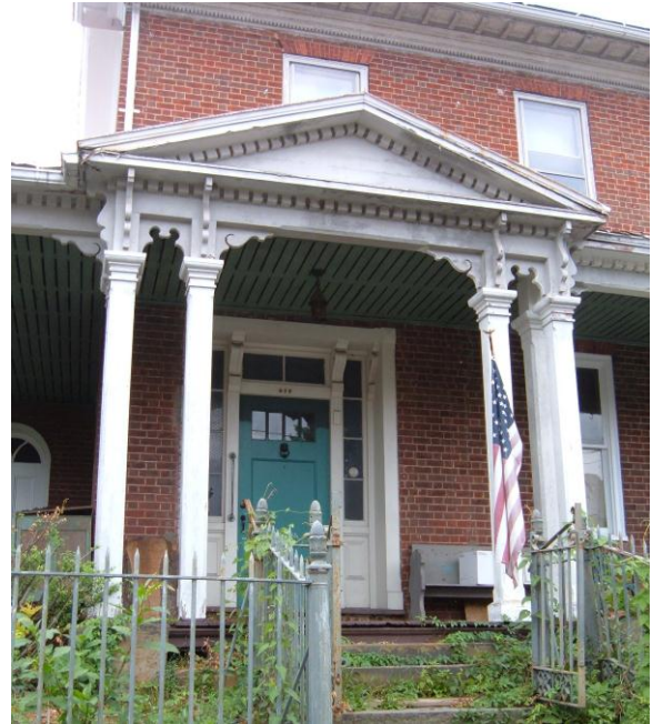
Italianate style porch at 917 Federal Street with square columns and eave brackets.
