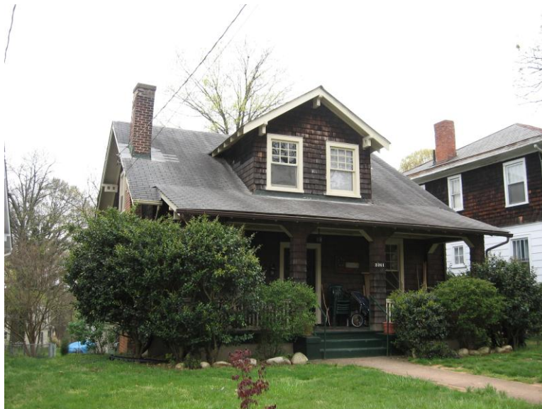
Shingled Craftsman dwelling at 2241 Rivermont Avenue.
