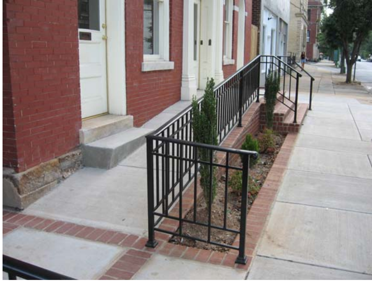
Appropriate handicap ramp at 1107 Church Street.
