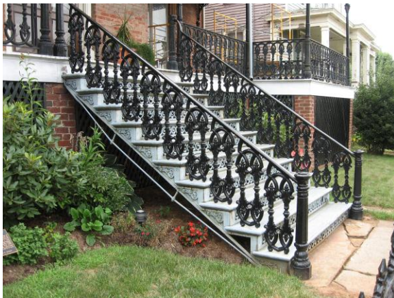
Original cast iron stairs should be preserved and maintained (602 Washington Street).
