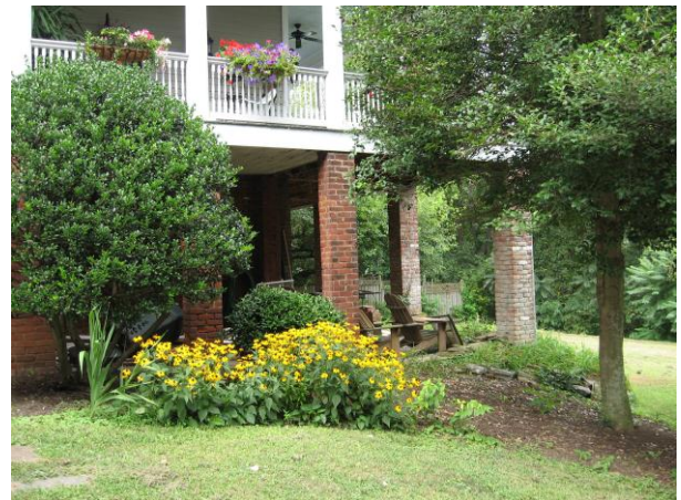
Brick pier foundations are often prominent features due to the steep slopes in the "Hill" districts (401 Washington Street).
