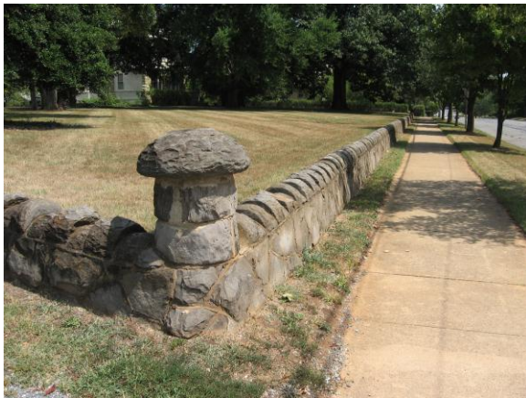
Original stone wall at 2024 Rivermont.
