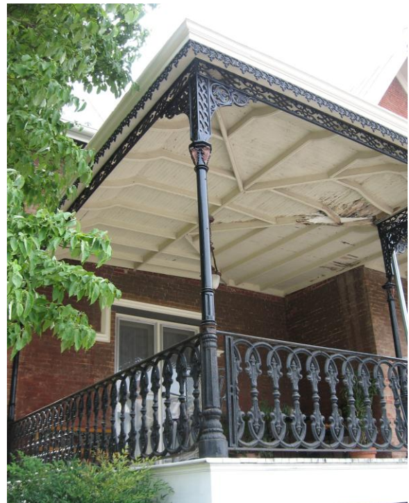
Cast iron porch columns are essential to defining a property's architectural character (602 Washington Street).
