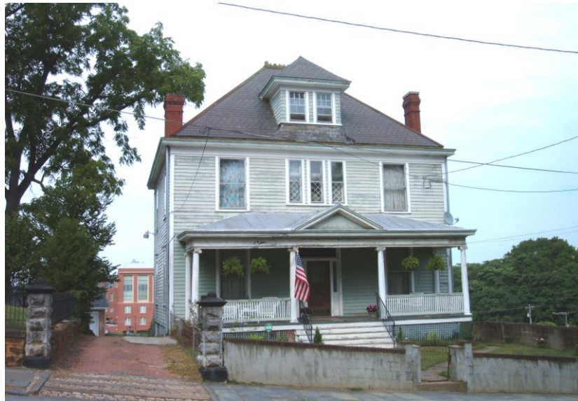
American Foursquare dwelling at 1112 Harrison Street.
