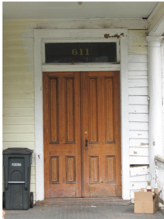
Original paneled wood doors at 611 Washington Street.
