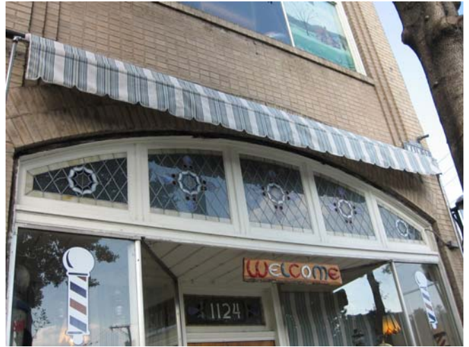
Retractable awnings are both appropriate and practical for storefronts (1124 Main Street).
