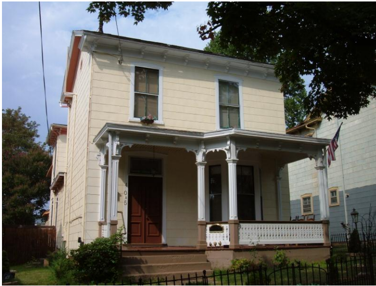
Side gable dwelling at 405 Harrison Street with milled columns.
