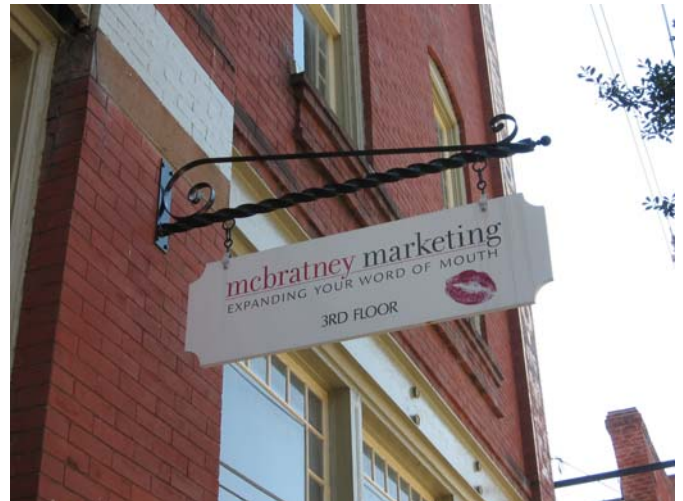
Projecting sign at 1022 Commerce Street.
