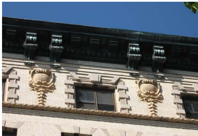
Preserve and maintain original sheet metal cornices (829 Main Street).
