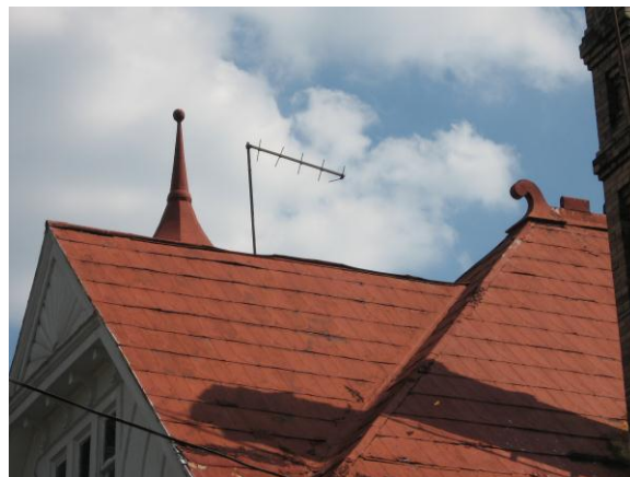
Original metal shingle roof at 429 Rivermont Avenue.
