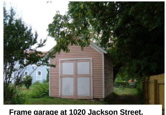
Frame garage at 1020 Jackson Street.
