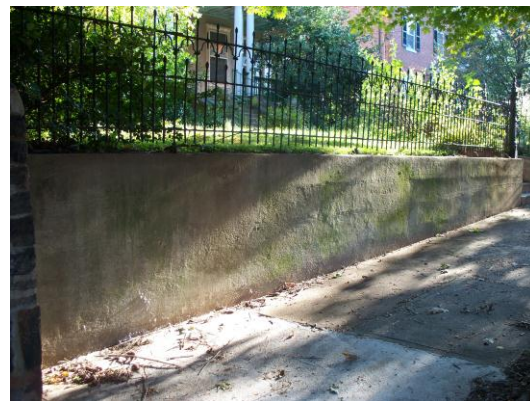
Concrete wall on Washington St.
