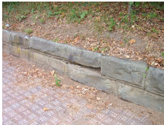
Stone retaining wall in the 900 block of Federal Street.
