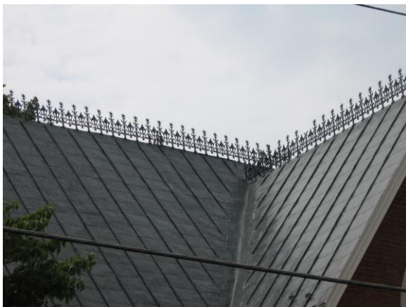
Original metal standing seam roofs should be maintained and repaired if needed (602 Washington Street).
