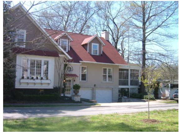
...and appropriately scaled rear addition.
