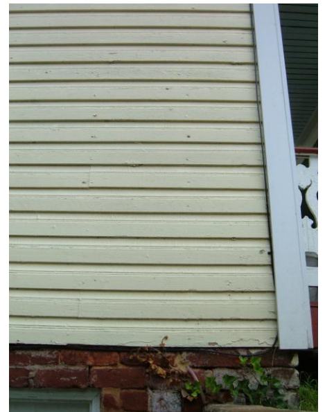
Original wood siding at 1000 Harrison Street.
