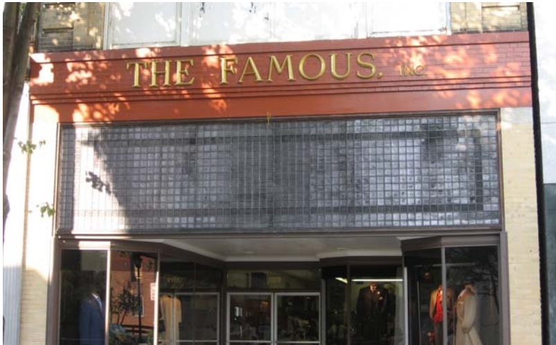
Original transom of "Luxfer" or prism glass at 1019 Main Street.
