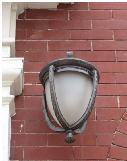
Appropriate new Colonial Revival influenced wall fixture at 1107 Church Street.
