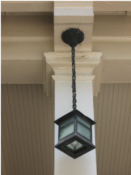
Preserve and maintain original light fixtures (2132 Rivermont).
