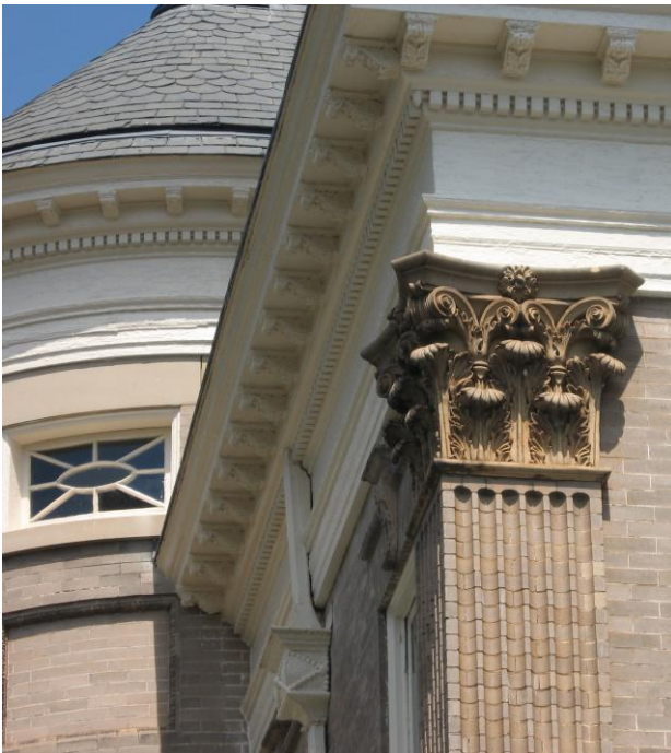
Preserve and maintain details such as terra cotta capitals (2024 Rivermont Avenue).
