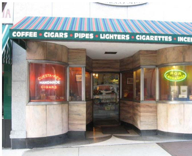
Storefronts which were rebuilt or remodeled in the 1930s and 1940s should be preserved such as this Art Moderne style storefront at 817 Main Street.
