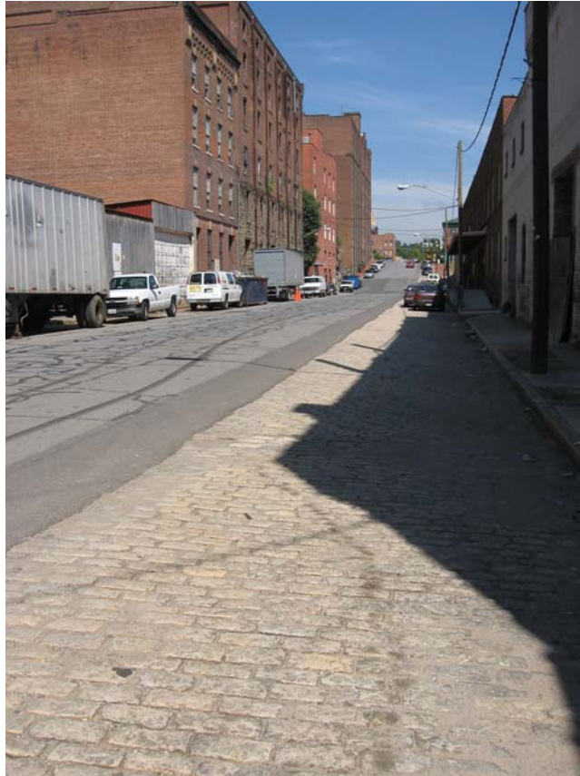
Streetscape in the 1000 Block of Jefferson Street showing the warehouse and manufacturing buildings of Lower Basin as well as a remaining section of cobblestone pavement.
