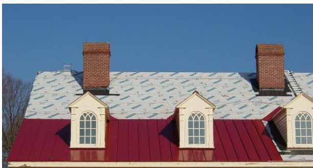
If replacement is necessary use a metal seam roof similar in dimensions, spacing and crimping as the original.
