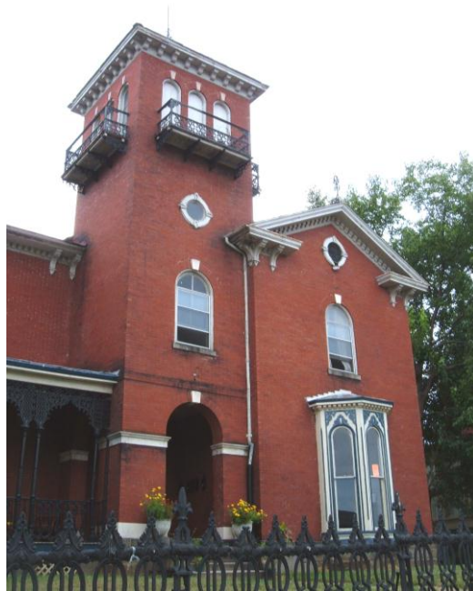
The James W. Watts House built in 1880 is Lynchburg's most notable example of an Italian Villa (1007 Court Street).
