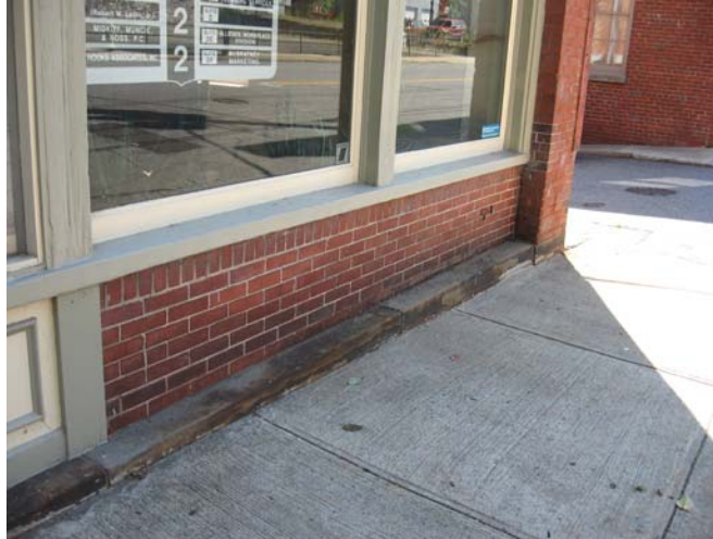
Original brick bulkhead at 1022 Commerce Street.
