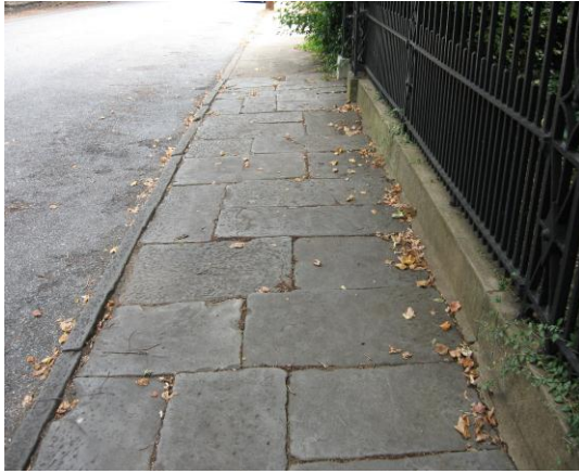
Stone sidewalk in the 500 block of Washington Street.
