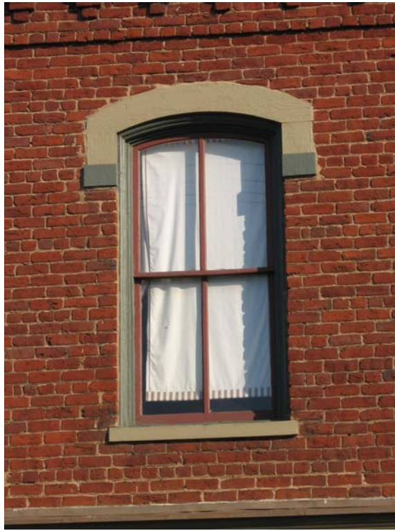
Preserve and maintain original windows (325 12 th Street).
