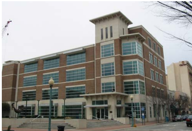
More contemporary in design, this new building is compatible in its materials, vertical divisions, and fenestration facing the street.
