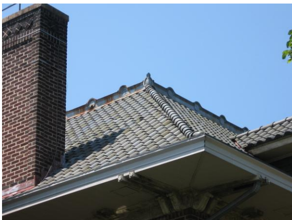
Original clay tile roof at 2701 Rivermont Avenue.
