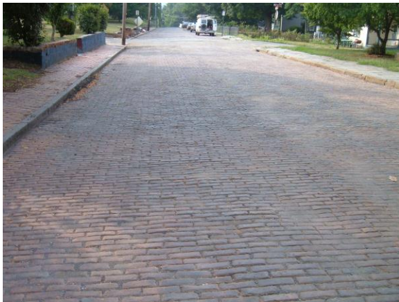
Restored brick surface on Cabell Street.
