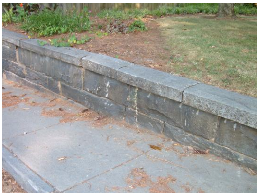
Stone retaining wall at 900 block of Federal Street
