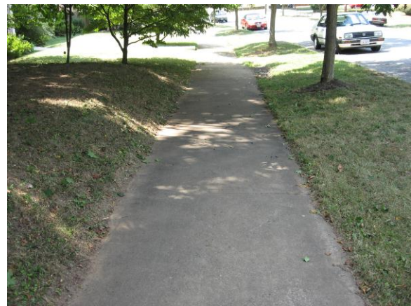
Concrete sidewalk on the 2200 block of Rivermont Avenue.
