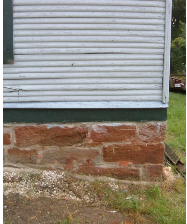
Preserve, maintain and repoint correctly original stone foundation materials (302 Cabell Street).
