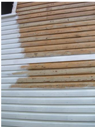
Removal of original paint and priming the wood surface helps to ensure a long lasting paint job (1102 Federal Street).
