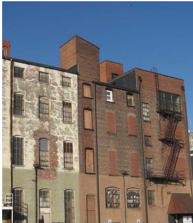
Gutters and downspouts at the rear of buildings along Main Street.
