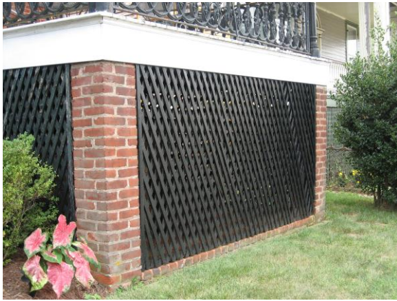
Lattice panels are appropriate and recommended for infill between brick pier foundations (602 Washington Street).
