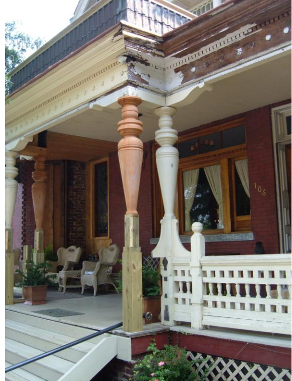
Porch column replacement to match the original at 106 Madison Street.
