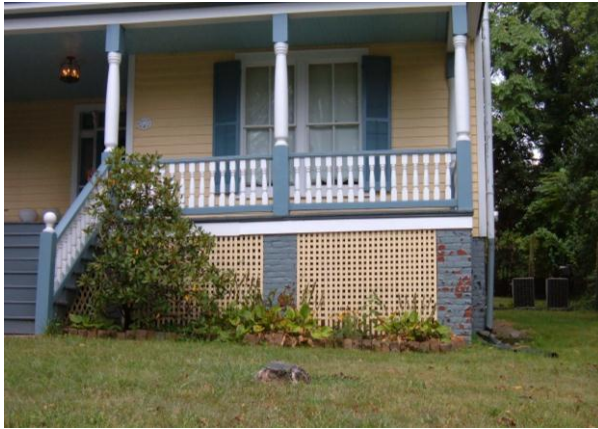
Appropriate lattice panels between brick piers (1015 Federal Street).
