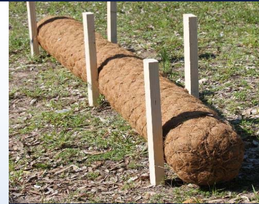
Erosion control matting and coir logs will stabilize stockpiles and slow run-off
