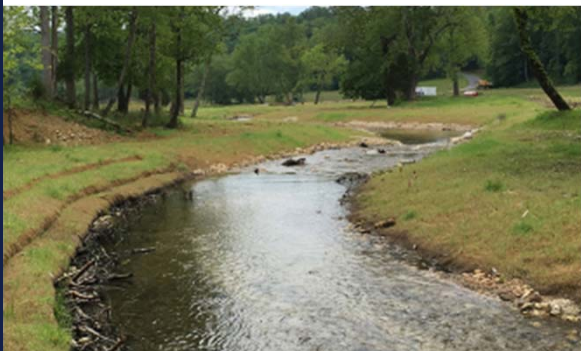
Toe wood bank protection
