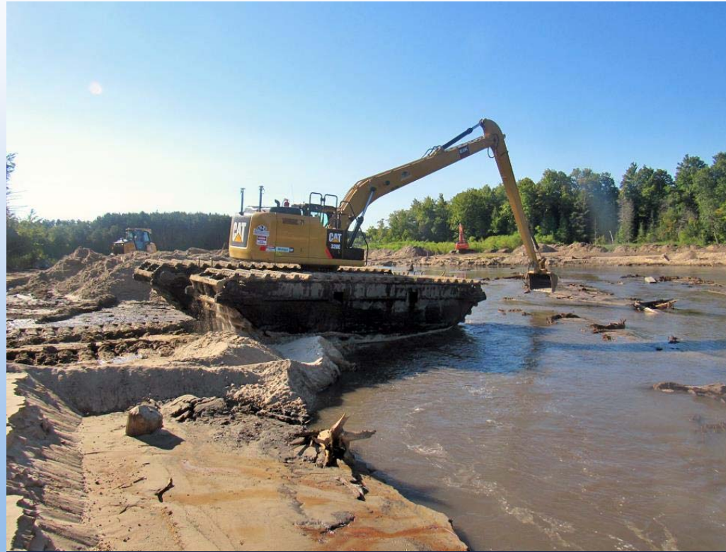
Impounded sediment will be removed by mechanical methods with specialized equipment
