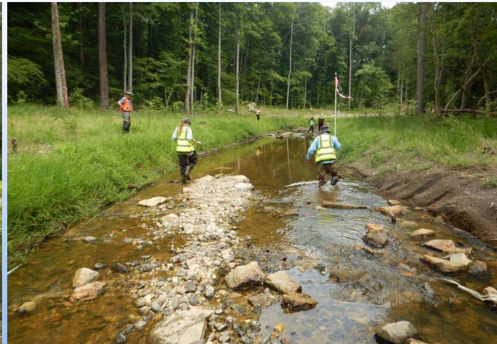
Construction operations will be observed by engineers specializing in stream restoration, sediment management, dam removal, and geotechnical engineering
