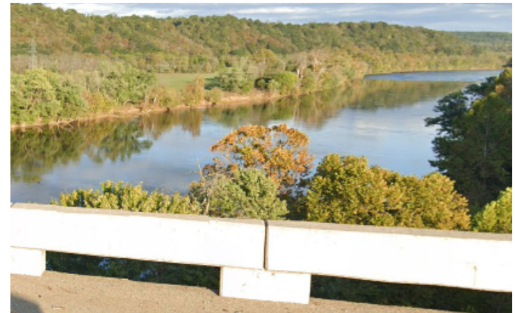
Above: Overlook project location Below: View from the Monocan Bridge Lynchburg, VA
