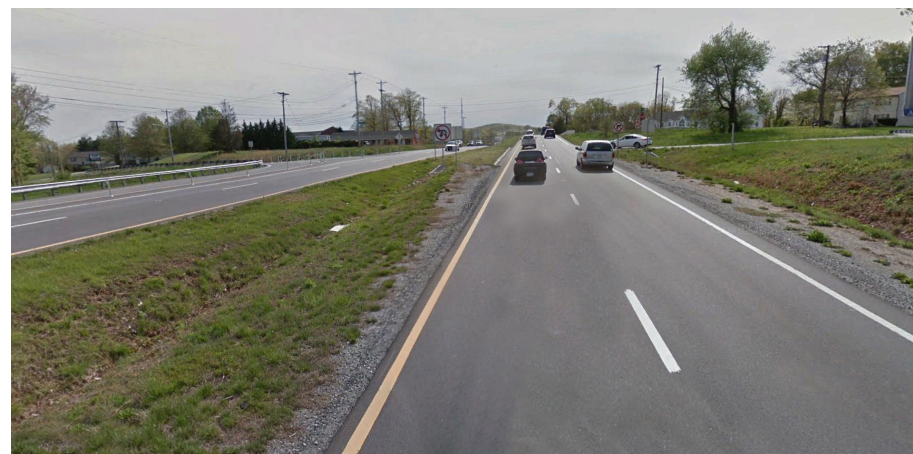
Existing conditions on U.S. Route 29/ U.S. 460 Bypass
