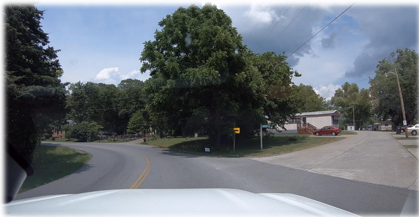
Figure 11 Sign Obscured by Trees
