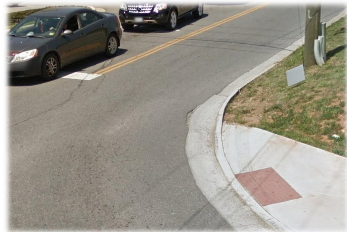
Figure 22 Northeast Corner of Lakeside Drive
