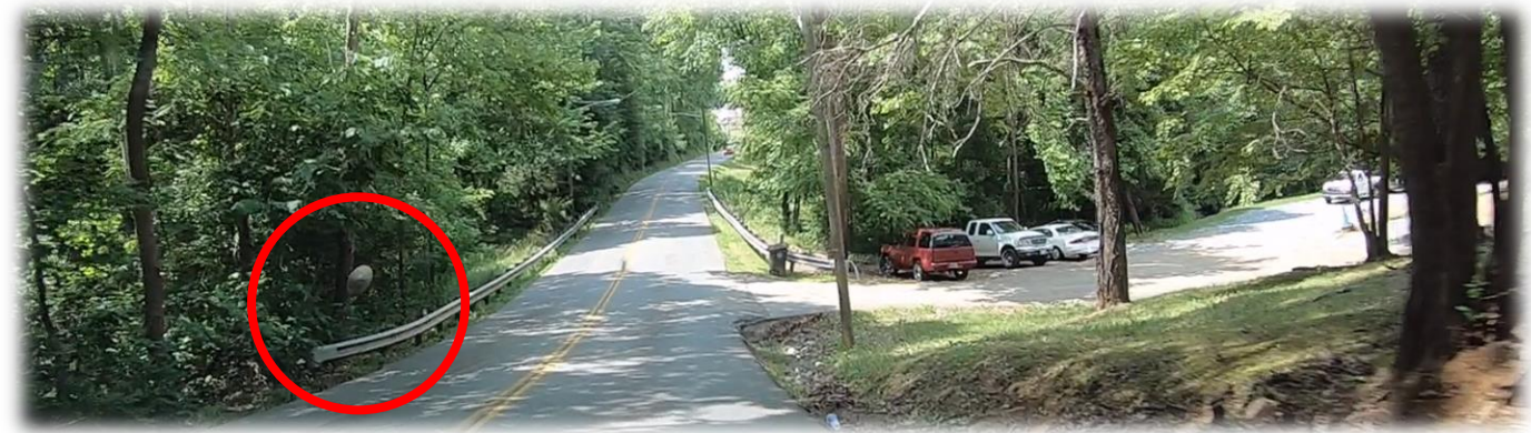
Figure 6 Convex Mirror for Sight Distance Issues at Private Entrance
