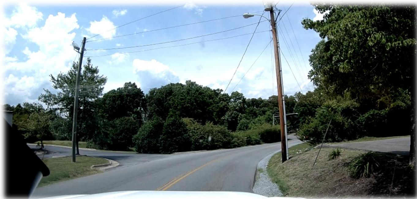
Figure 12 Gravel Fill for Recurrent Overrunning of Road
