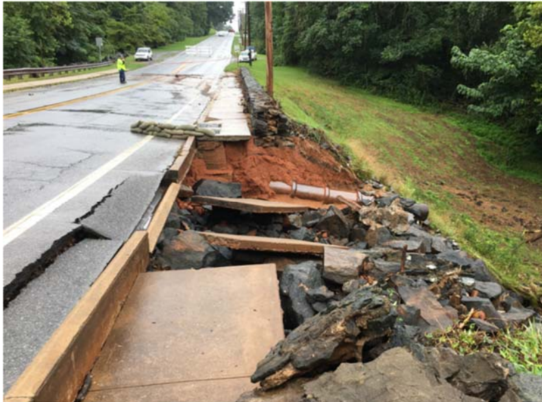
College Lake Dam
