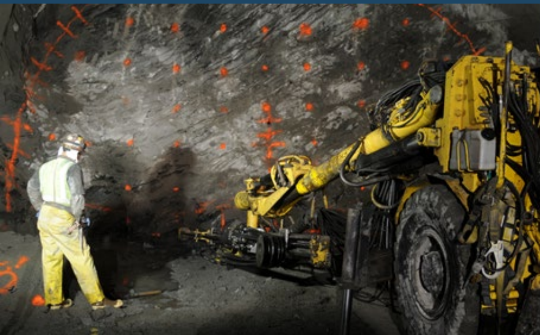
Tunnel excavation method will be drill & blast
