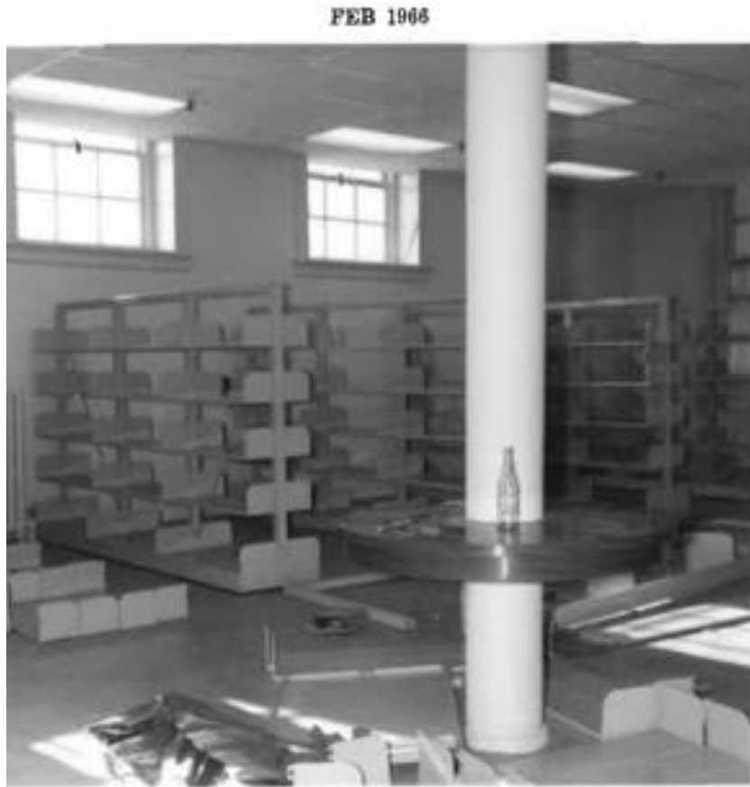
Library shelving while under construction in 1966. Same shelving is currently in use today.
