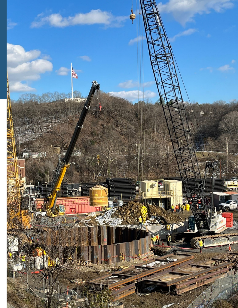
LYHBeyond, the Blackwater CSO Tunnel project, began construction in FY 2025.
