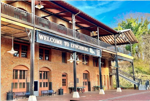
Kemper Street Station
