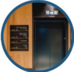
New Elevator and Vestibule
