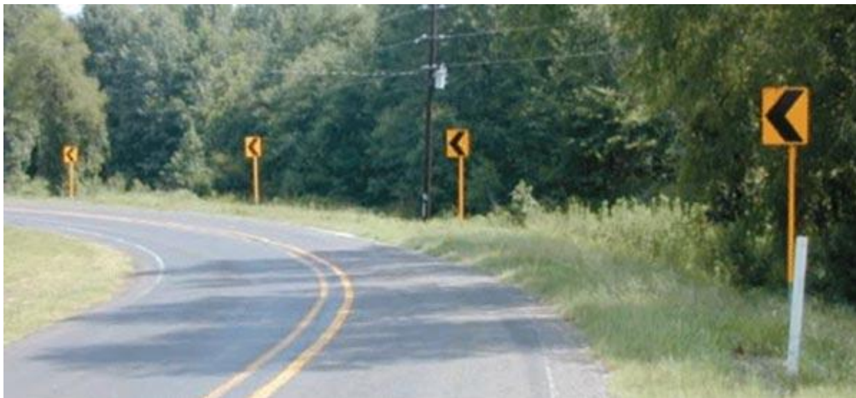
Figure 22: Curve Delineation. Source: FHWA
