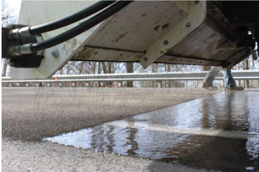
Figure 24: High-Friction Surface Treatment. Source: FHWA
