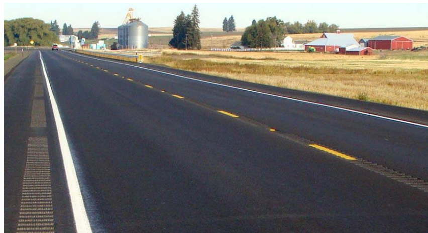
Figure 23: Edge line and Centerline Treatments. Source: FHWA.
