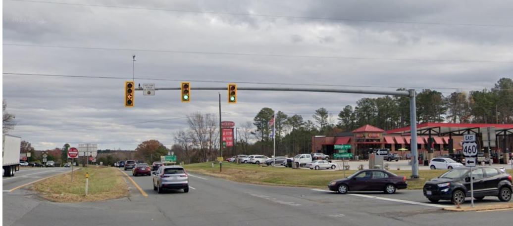
Figure 28: Flashing Yellow Arrows. Source: Google Maps
