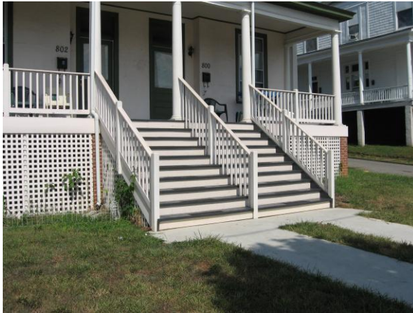
Rebuilt wood stair at 800-802 Rivermont Avenue.
