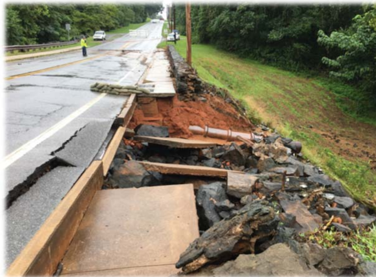
College Lake Dam
