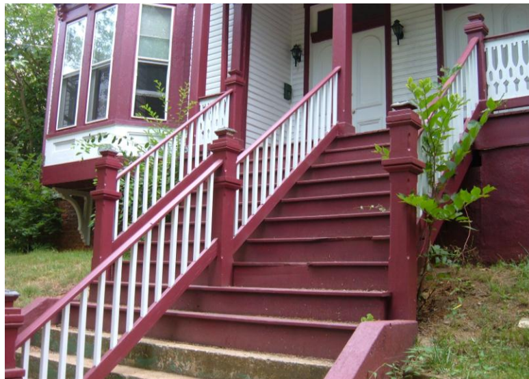
Appropriate rebuilt staircase at 202-204 Harrison Street.
