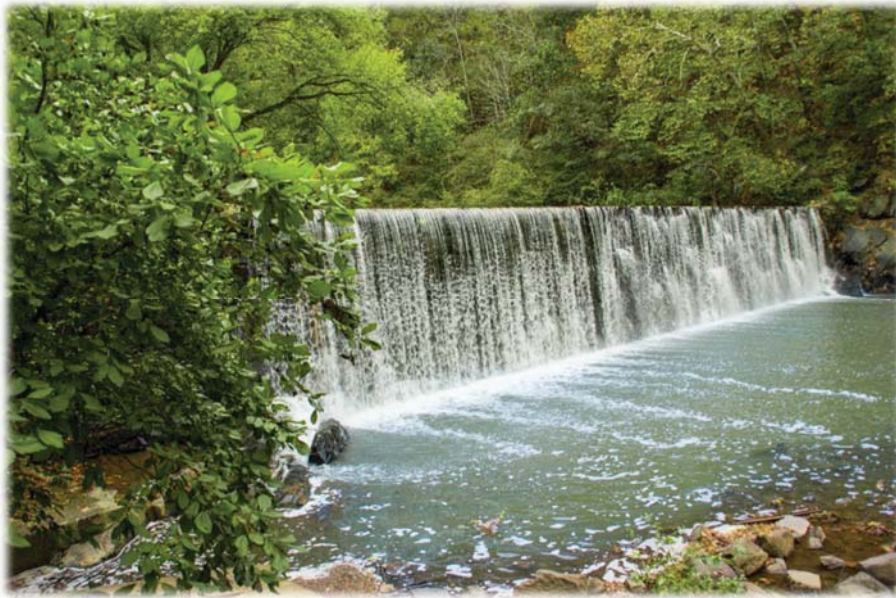
Hollins Mill Dam
