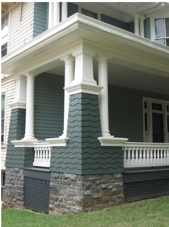
Tapered Craftsman style porch columns at 1314 Clay Street.
