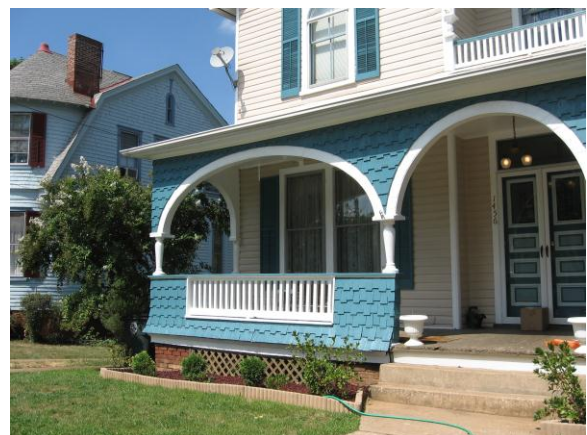
Queen Anne style porch with milled columns and wood shingle railing at 1456 Rivermont Avenue.
