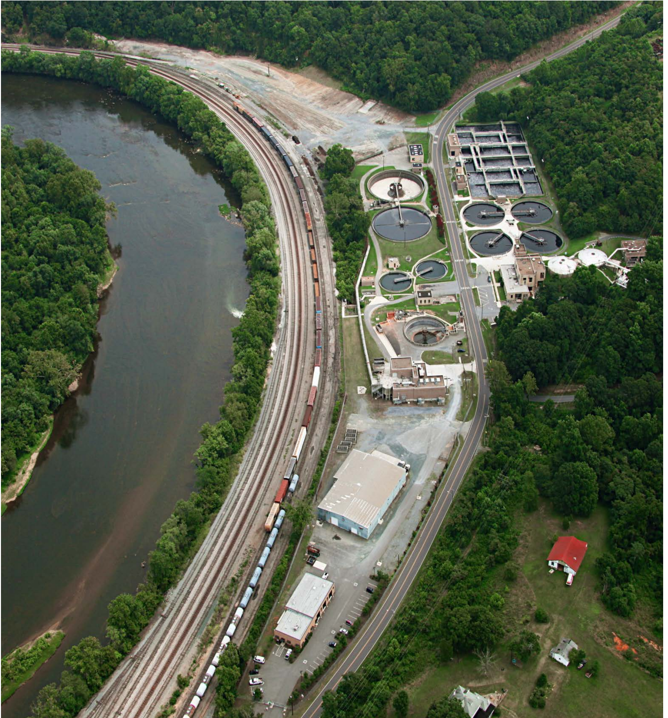
Lynchburg Regional Wastewater Treatment Plant
