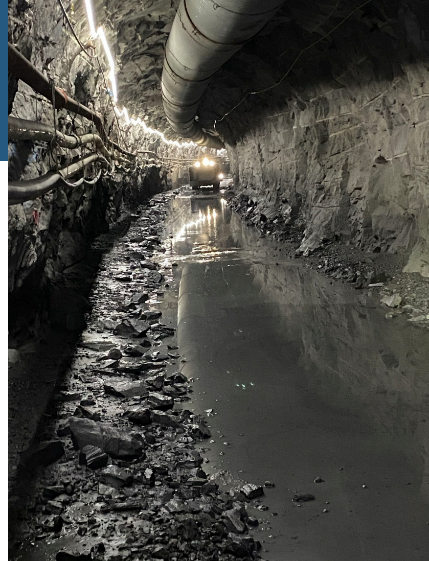
Blackwater CSO Tunnel Excavation
