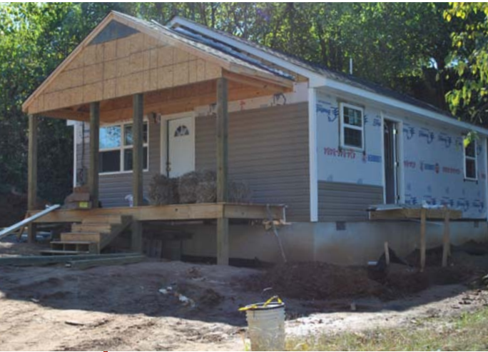
Substantially reconstructed home during construction within the project area.
