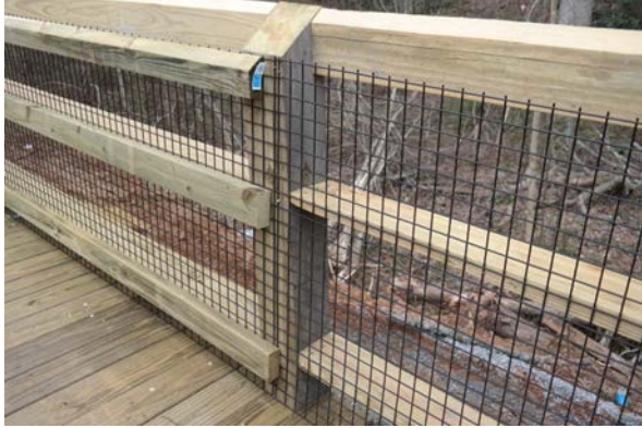
Photo No. 7: Fencing
