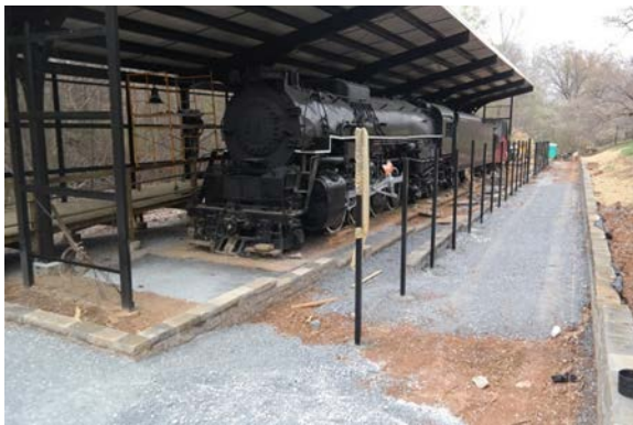
Photo No. 9: Installing Fencing
