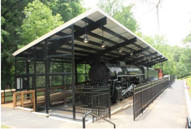
Photo No. 4: Train Shed after Grand Opening
