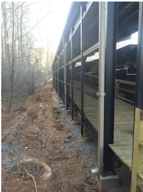
Photo No. 8: Constructing Swale
