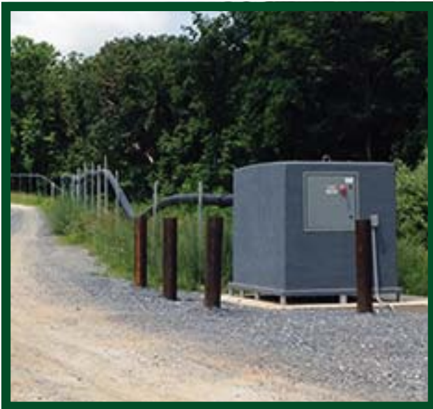
Vapor-Phase Perimeter Odor Mitigation System
