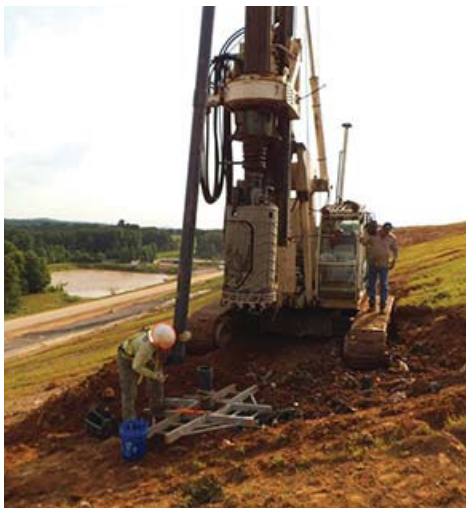
Landfill gas extraction well
