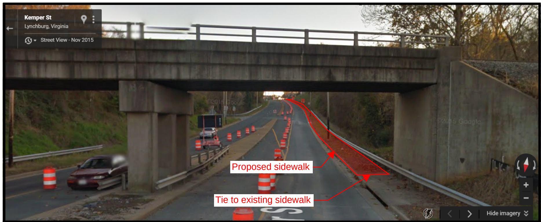
Kemper Street at Norfolk Southern Bridge, Start of project
