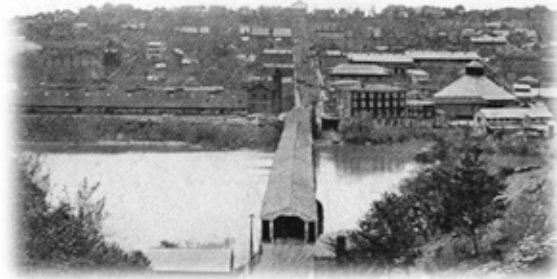
Covered Bridge at 9 th Street
