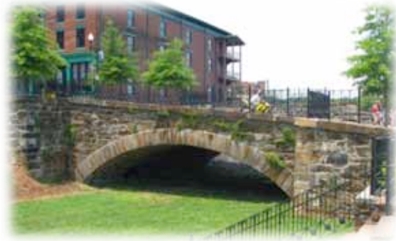
Existing Conditions – 9 th Street Kanawha Canal Bridge
