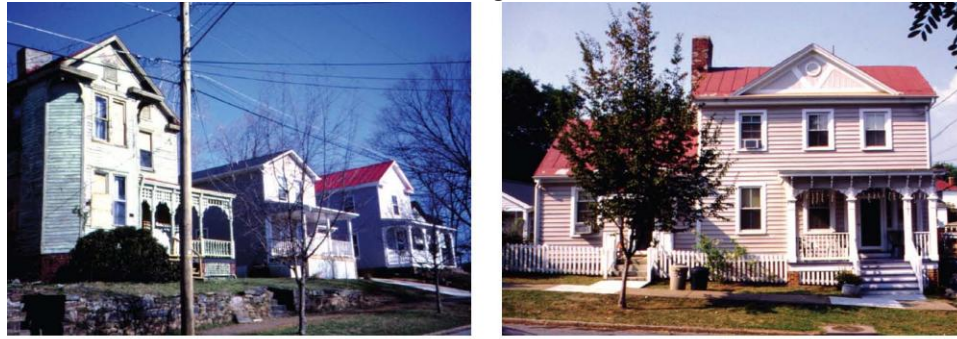
Illustrative, Rehabilitated Neighborhood Conservation Area 2002
