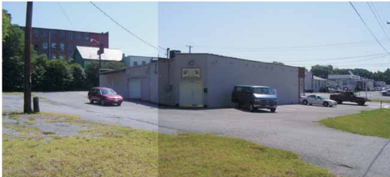
1713 12th Street 1110 Kemper Street
