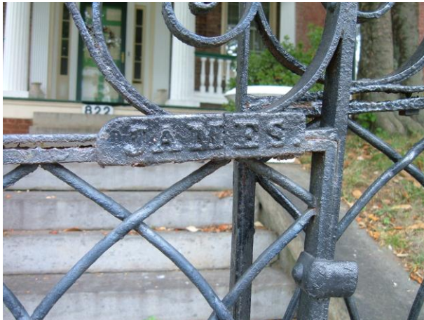
Cast iron fence with manufacturer's plate at 822 Federal Street.
