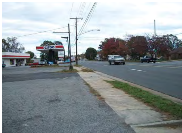
UNEVEN SIDEWALK WITH MULTIPLE CURBCUTS ON CAMPBELL AVENUE AT CITGO STATION
