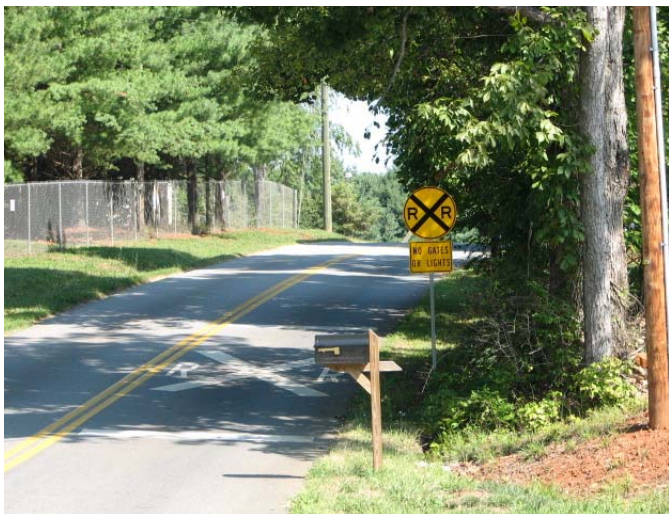
Advanced warning signs coming from south. Note vertical curvature of road that obscures crossing.
