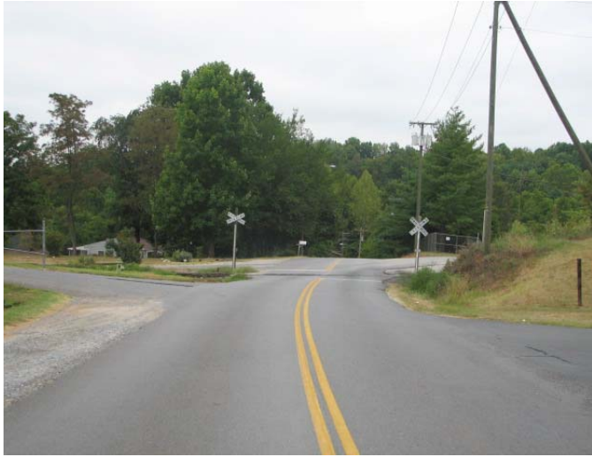
Looking south showing hill obstruction to the west (right of crossing). Note rail crossing almost disappears due to topography issues.
