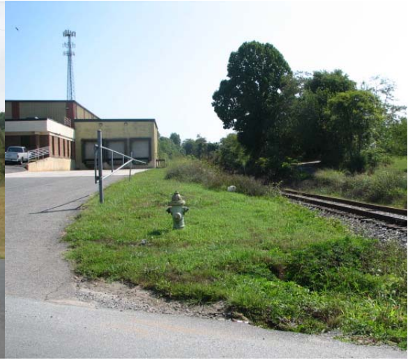
Looking east at sunken rail tracks that also blocks sight distance of train. This photo was taken at stop bar at driver's height.
