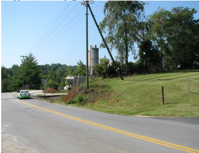
Another view showing hill to west blocking entire view of train.
