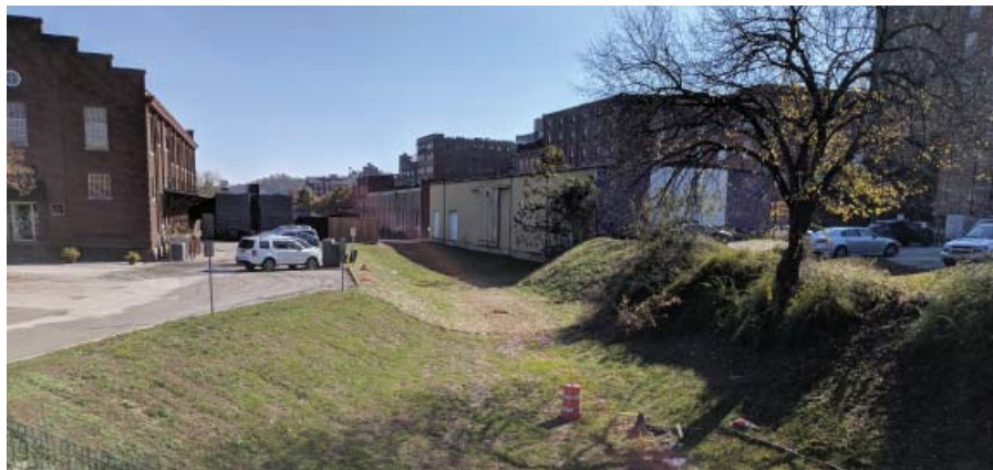
Canal Park - Existing Conditions, 9th Street Bridge
