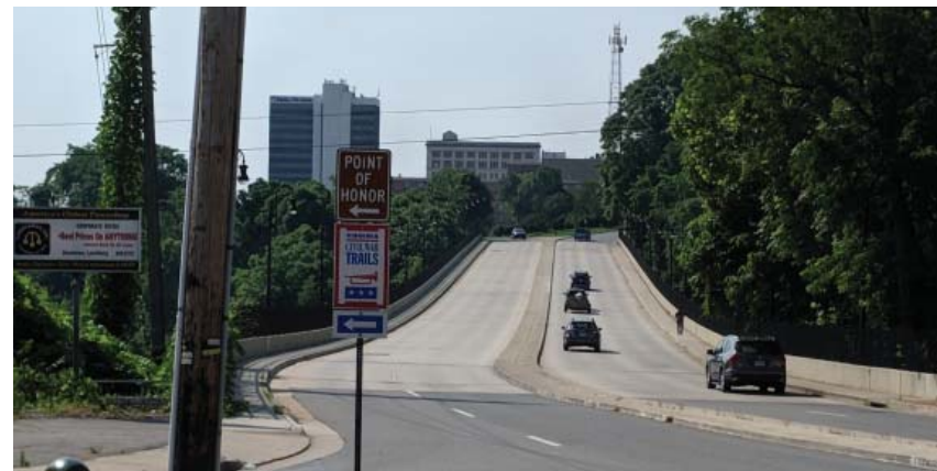
Rivermont Bridge in 2018
