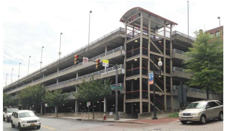
901 Commerce Street - Existing Parking Structure
