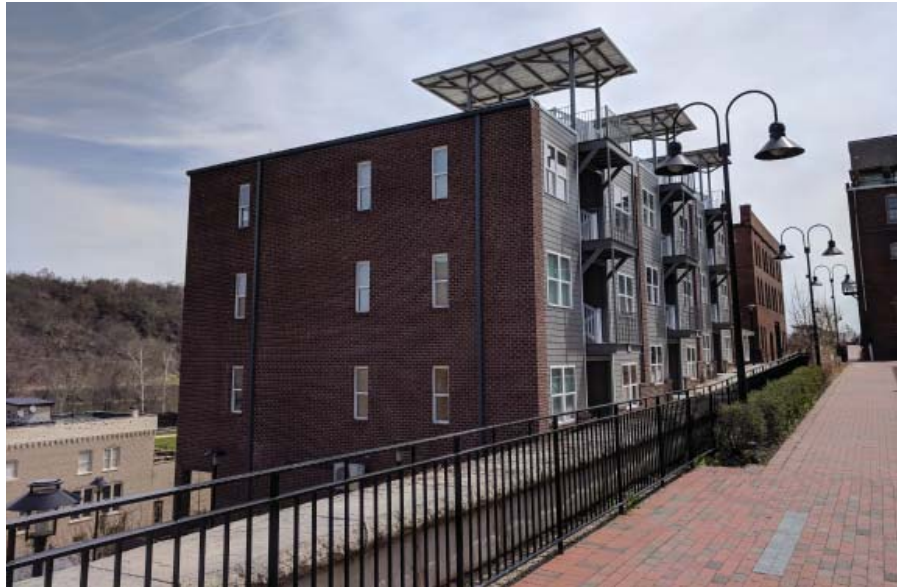
51 11th Street Lofts on the Lower Bluffwalk.
