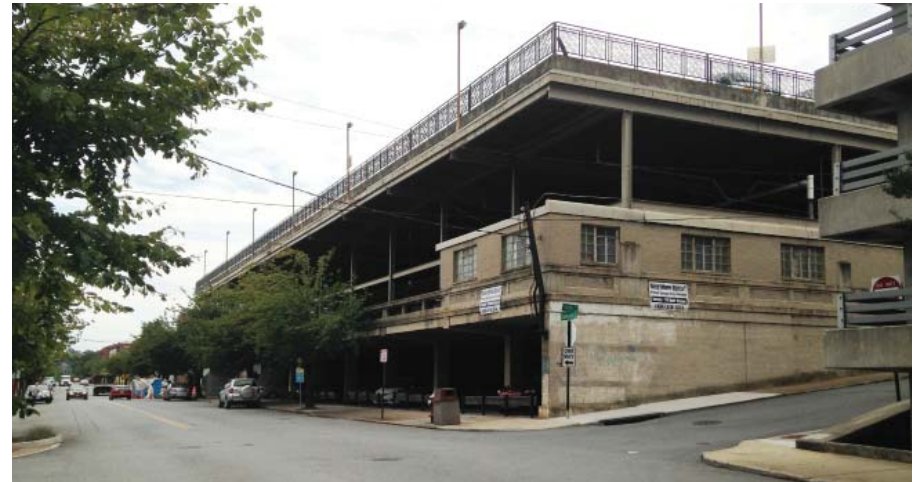
1001 Commerce Street - Historic Parking Structure
