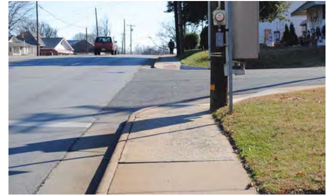
SIDWALK ON CAMPBELL AVENUE OFTEN LACKS BUFFERS AND CROSSWALKS
