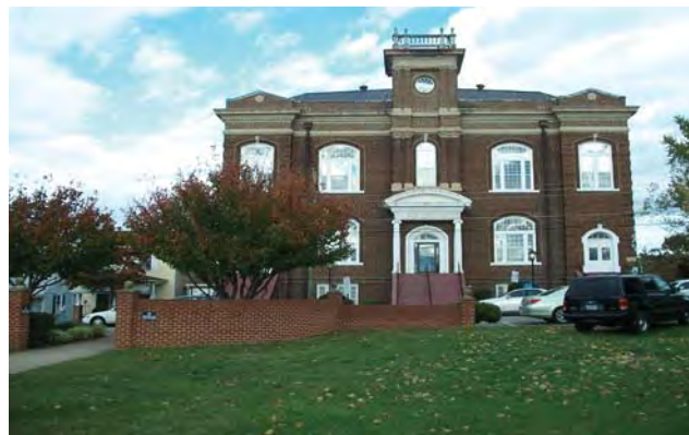
HISTORIC HUMBLER HALL ON THE VUL CAMPUS
