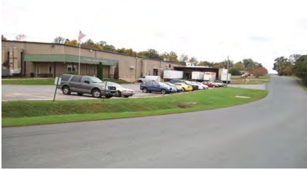
LYNCHBURG SHELTERED INDUSTRIES, A TYPICAL INDUSTRIAL USE IN THE ODD FELLOWS ROAD AREA
