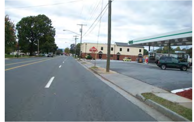
TYPICAL COMMERCIAL SEGMENT OF CAMPBELL AVENUE
