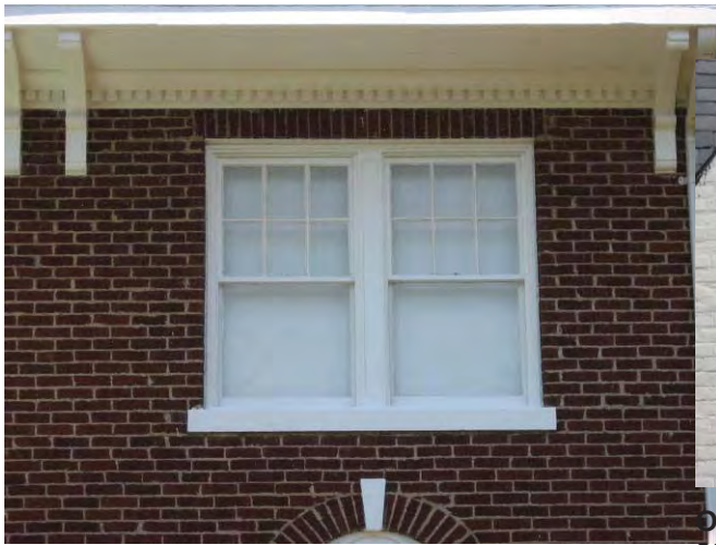
Preserve and maintain original historic windows such as six-over-one wood sash (2308 Rivermont).
