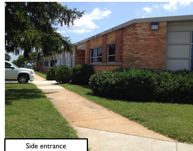
Sidewalk to side entrance
