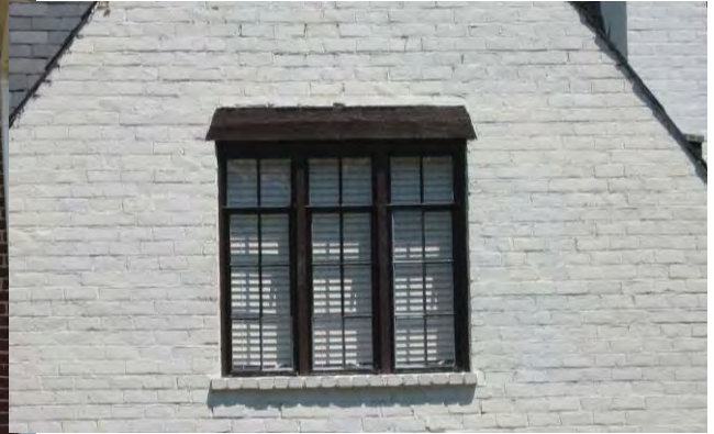
Original steel casement windows of the 20 th century should also be repaired as needed and retained.
