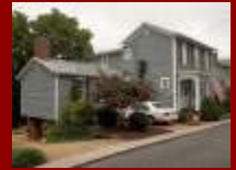
City's First Rehab at 507 13 TH ST [1984]
