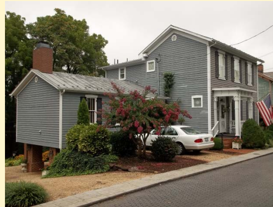
City's First Rehab at 507 13 TH ST [1984]
