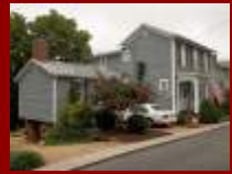
City's First Rehab at 507 13 TH ST [1984]
