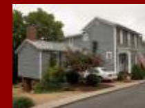
City's First Rehab at 507 13 TH ST [1984]
