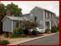
City's First Rehab at 507 13 TH ST [1984]
