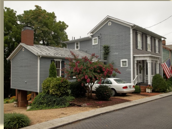
City's First Rehab at 507 13 TH ST [1984]
