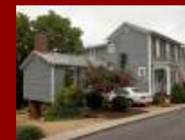
City's First Rehab at 507 13 TH ST [1984]
