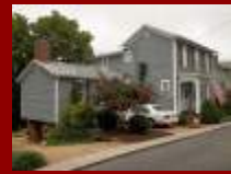
City's First Rehab at 507 13 TH ST [1984]
