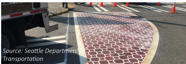
Painted curb extensions/bump outs slow traffic and narrow pedestrian crossings.
