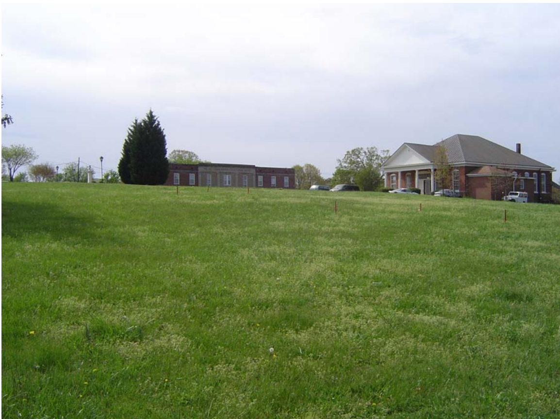
View from Railroad Tracks
