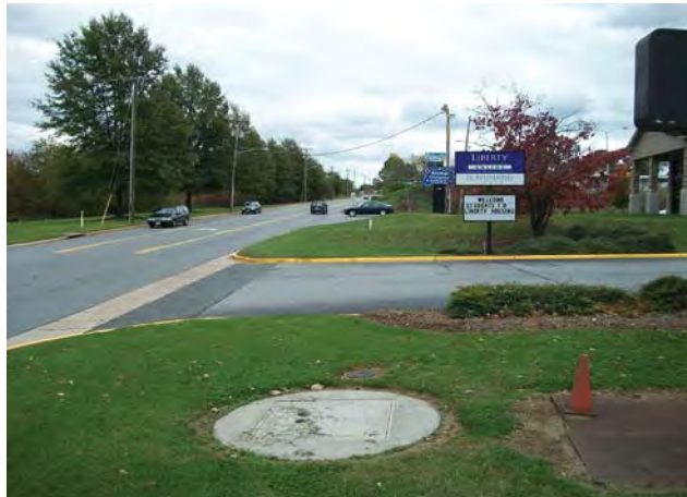
TYPICAL COMMERCIAL SEGMENT OF ODD FELLOWS ROAD
