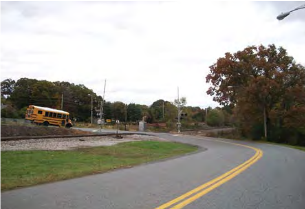
AT GRADE RAILROAD CROSSING ON MAYFLOWER DRIVE
