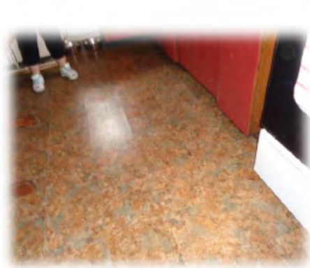
Floor after repair
