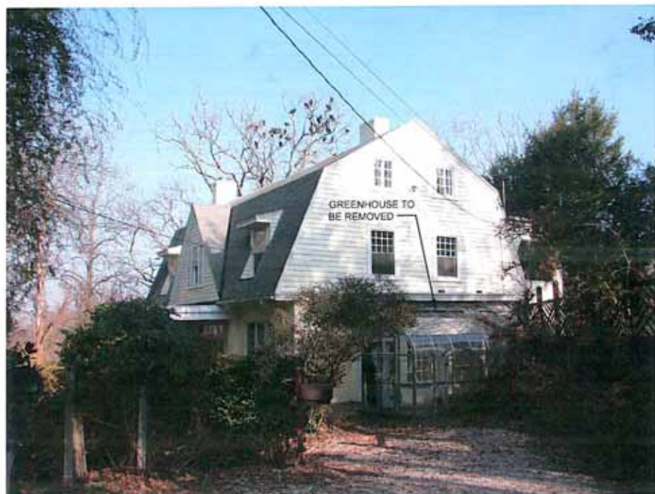
A VIEW OF SOUTHWEST (GUEST ENTRY) SIDE
