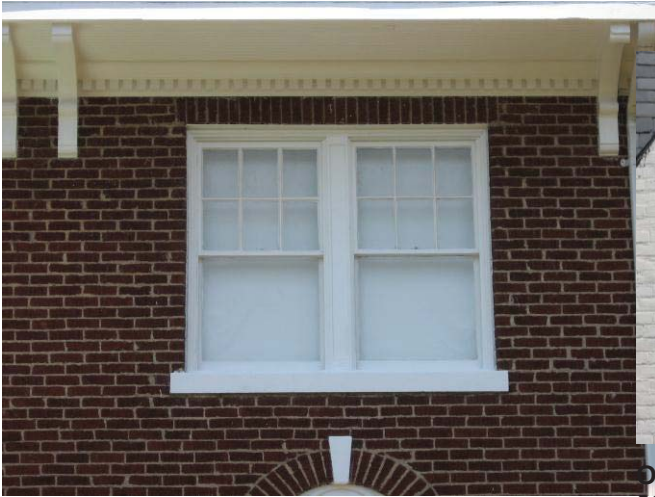
Preserve and maintain original historic windows such as six-over-one wood sash (2308 Rivermont).
