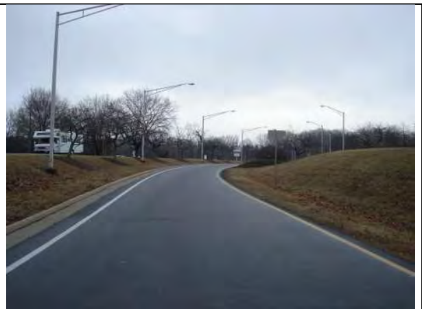
Looking north along Southbound Off Ramp near Candler Mountain Road
